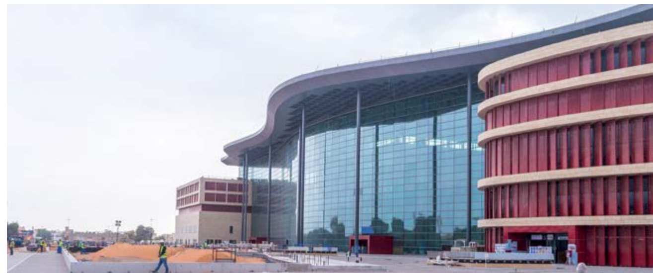
Al Ain Hospital, Abu Dhabi (United Arab Emirates)
