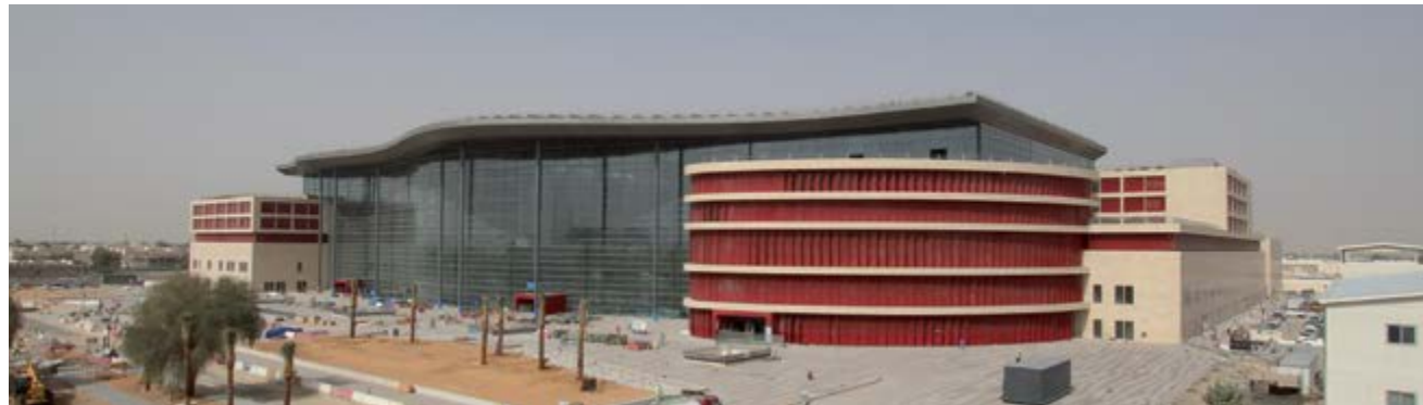
Al Ain Hospital, Abu Dhabi (United Arab Emirates)
