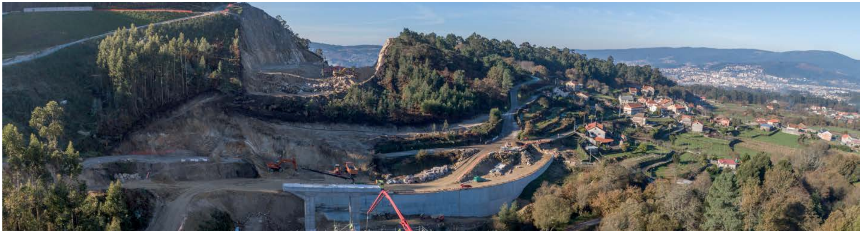
Stretch Vilaboa - A Ermida of the future Highway A-57, Pontevedra
