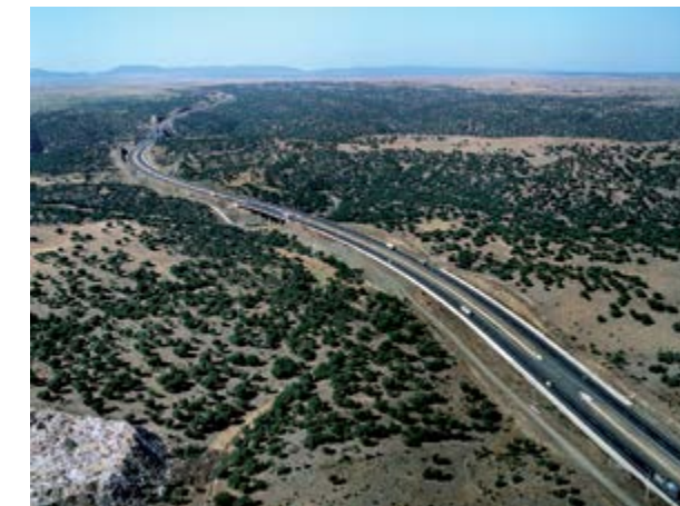
Road maintenance on State roads on sector CC-3 Caceres
