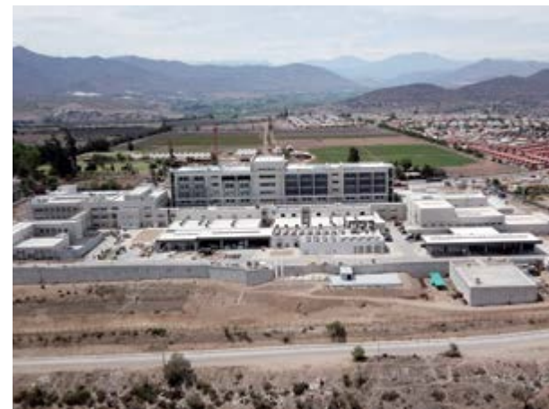
Hospital of Ovalle (Chile)
