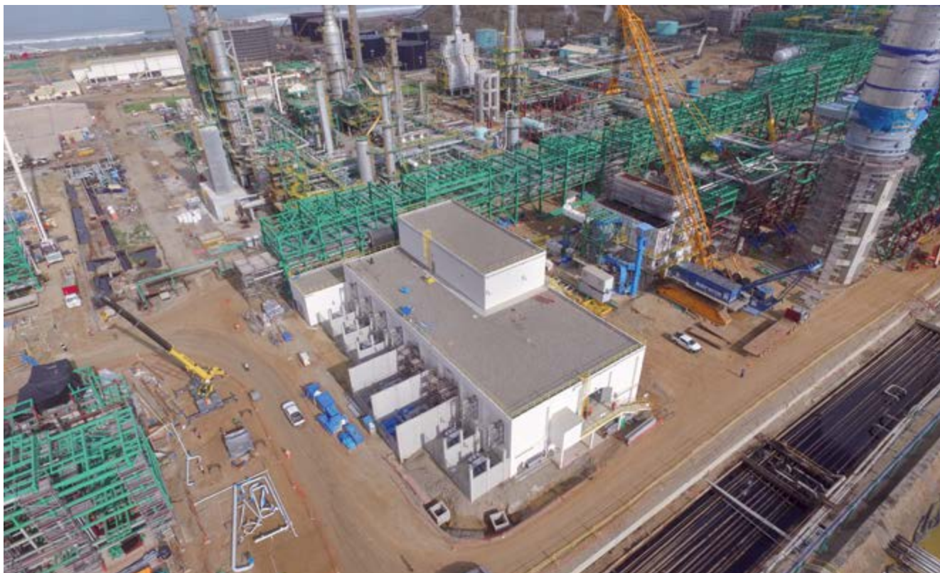
Control building and Electrical substations. Refinery Talara - Piura (Peru)
