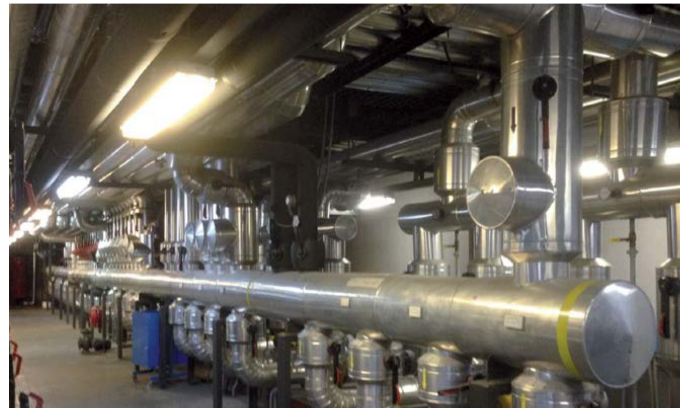
Adaptation of Central Cold / Heat plant in the building Corporación de Radio Television Española in Prado del Rey, Madrid (Spain)
