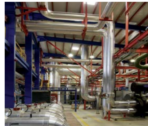
Power supplier of the first particle accelerator synchrotron in Spain and south western Europe: Alba Synchrotron.
