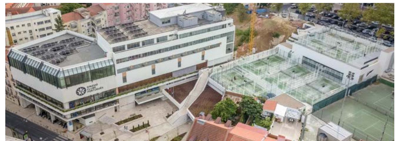
Enlargement and new underground car park spaces at Gimnasio Clube Português of Lisbon. (Portugal)
