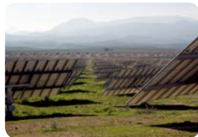
PV Solar Farm in < Alcaudete, Jaén - pag 84
