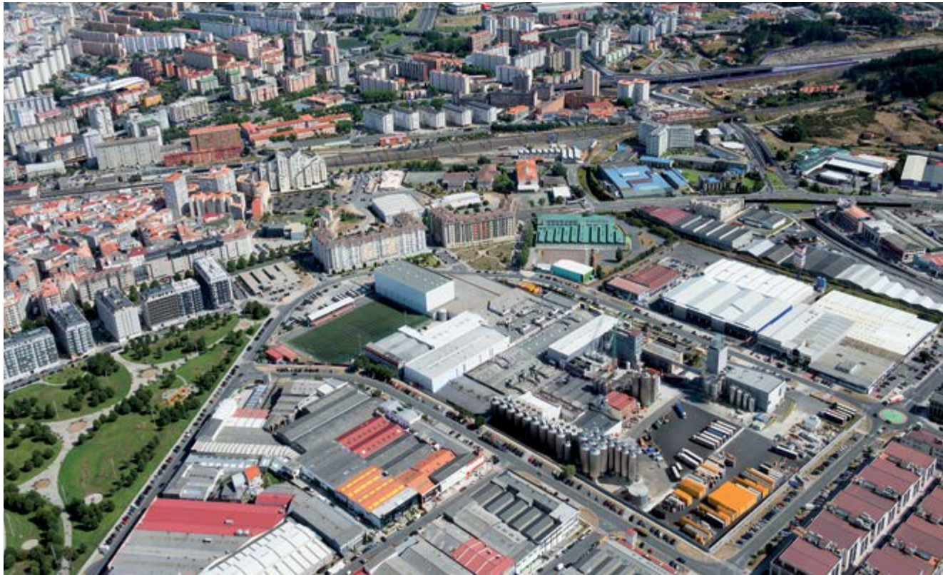
Enlargement and remodelling of the Estrella Galicia factory in A Coruña (Spain)
