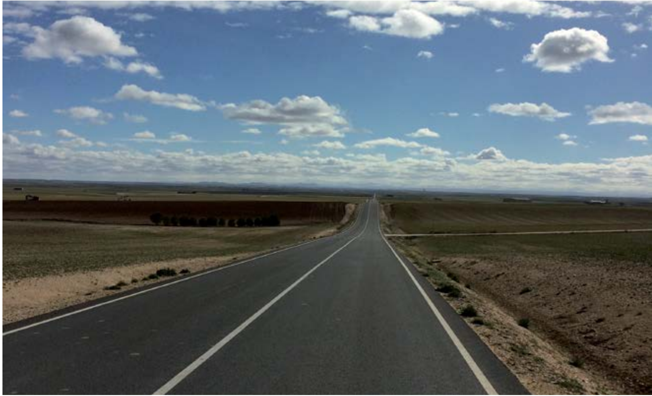
Reinforcement and replacement of road surface at SA-801 from Peñaranda de Bracamonte to CL-605, Salamanca (Spain)
