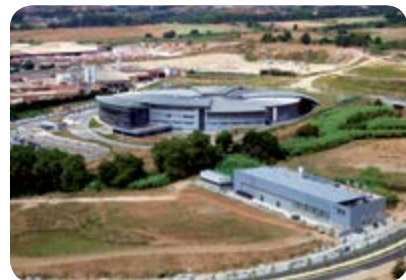
> District Heating and Cooling Poligeneration Power Plant ST-4 in Cerdanyola del Vallés, Barcelona - pag 82
