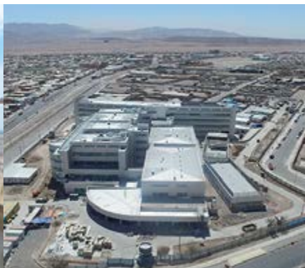
Carlos Cisternas Hospital, Calama (Chile)
