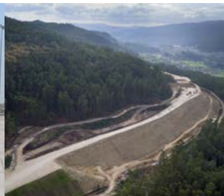
Stretch Vilaboa - A Ermida of the future Highway A-57, Pontevedra (Spain)
