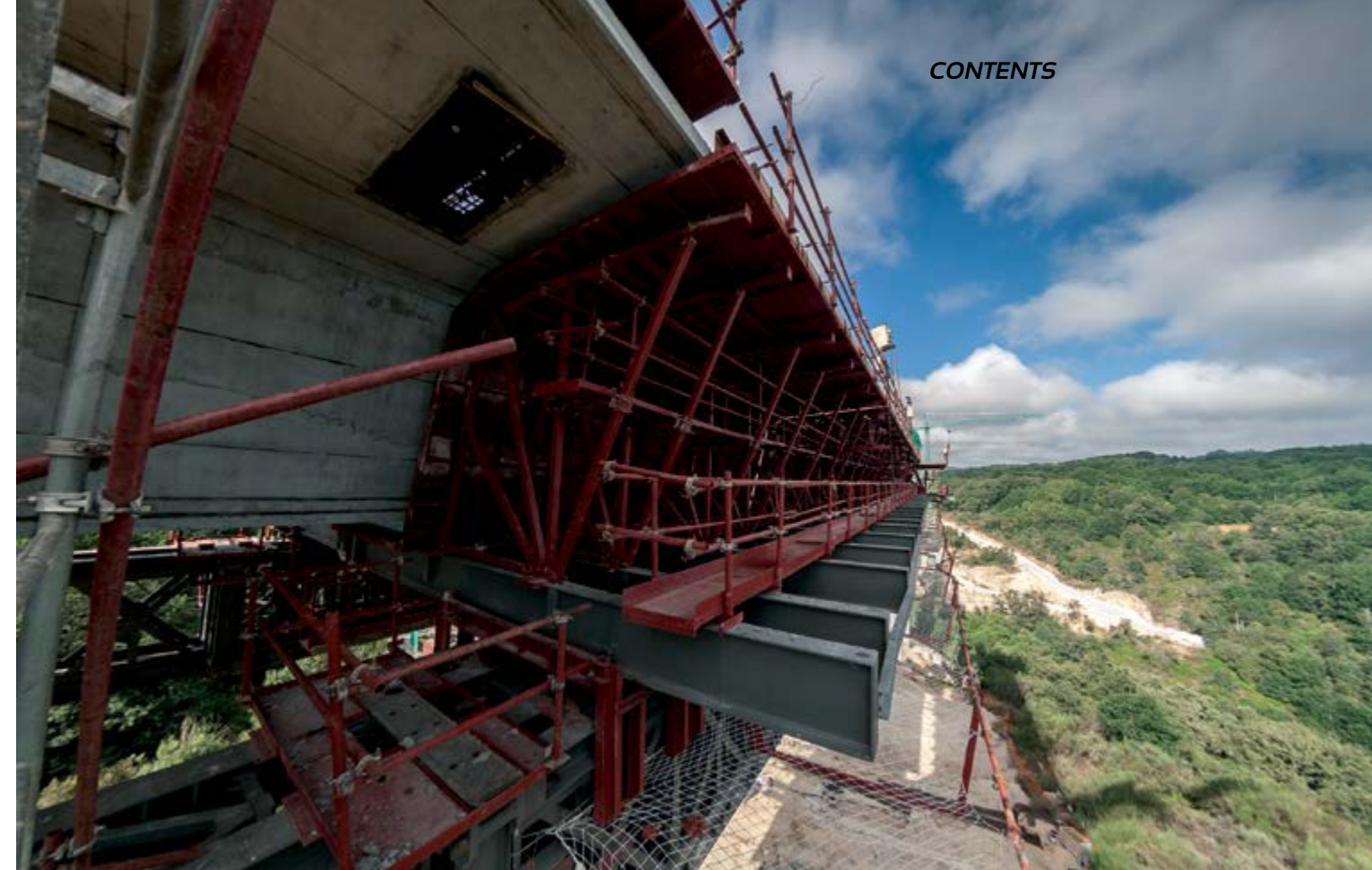
Stretch Miaman - Ponte Ambia (Orense). Spanish High Speed Railway Line AVE Madrid - Galicia (Spain)
