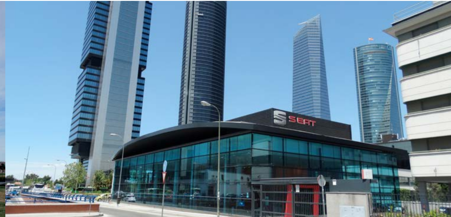
Refurbishment SEAT dealers at 278 Castellana St., Madrid (Spain)
