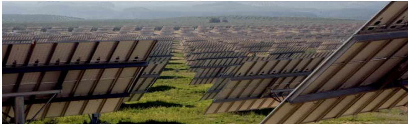
5.4 MW PV solar plant in Alcaudete, Jaen (Spain)
