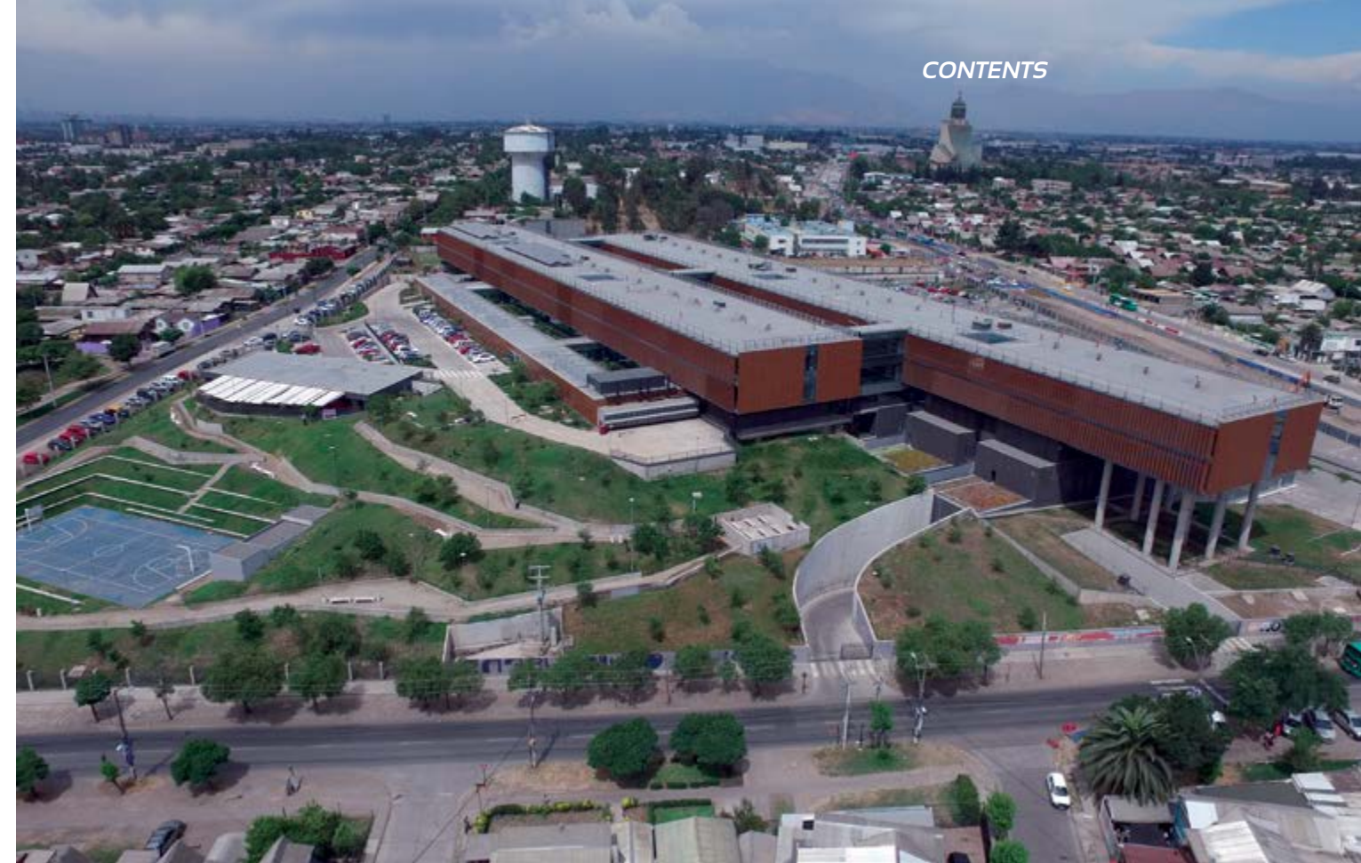
El Carmen Dr. Luis Valentin Ferrada Hospital of Maipu, Santiago de Chile. Engineering and project GSJ Solutions /Execution SANJOSE Constructora
