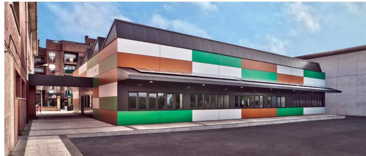
Refurbishment of the Secondary Institute of Zumaia BHI, Guipuzcoa (Spain)
