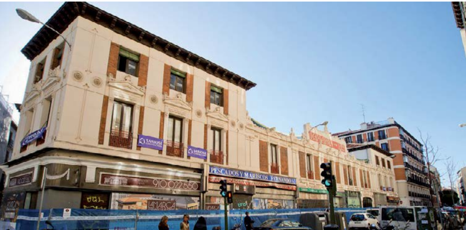
Lamarca housing building at Fernando VI St., Madrid (Spain)
