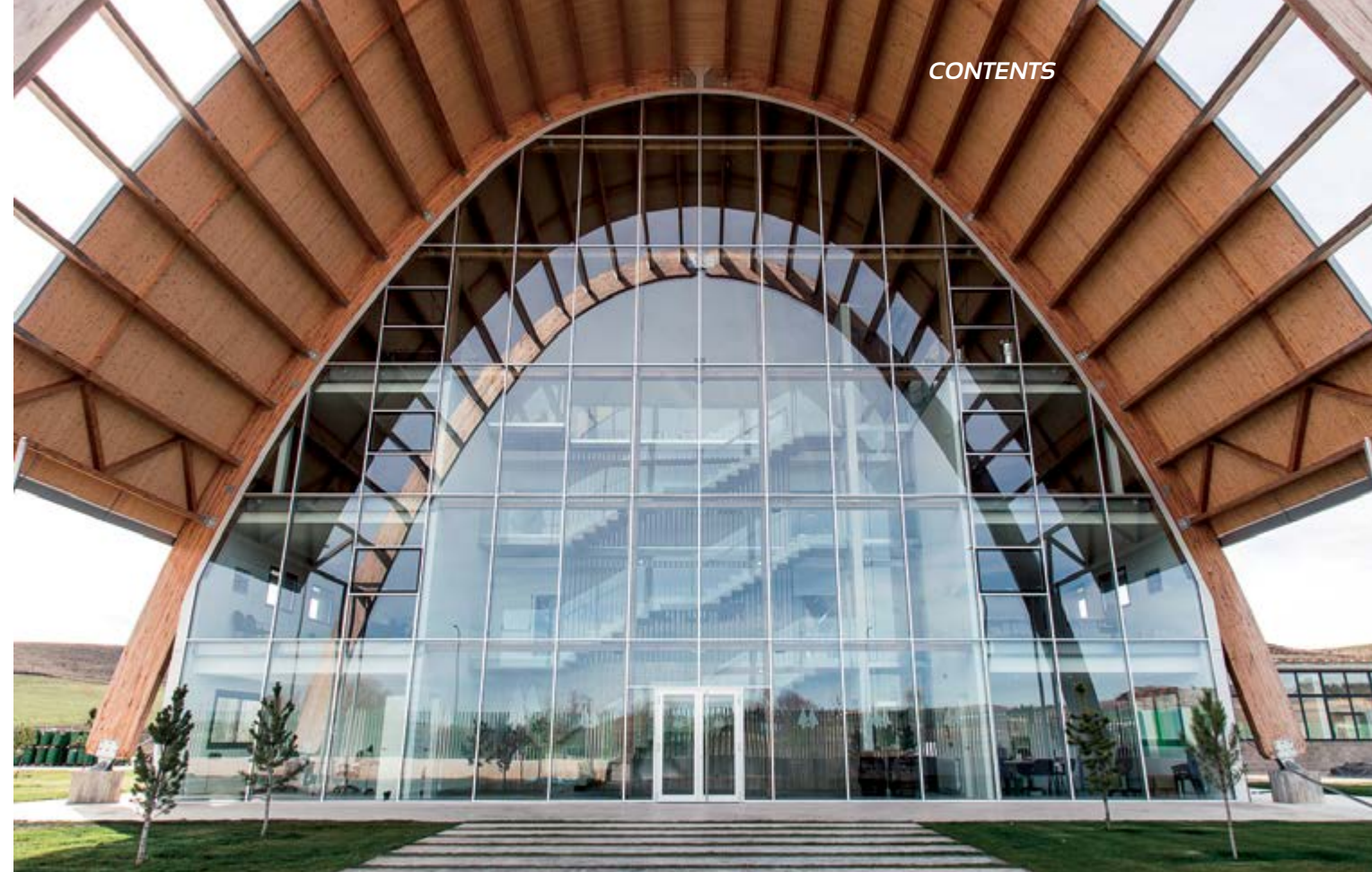
Building of the plant for the distillation of resin in Almazan, Soria (Spain)
