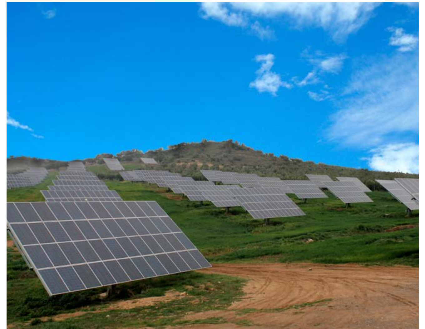
PV solar farm in Alcaudete, Jaén (5,4 MW). Engineering and project GSJ Solutions / Execution SANJOSE Constructora
