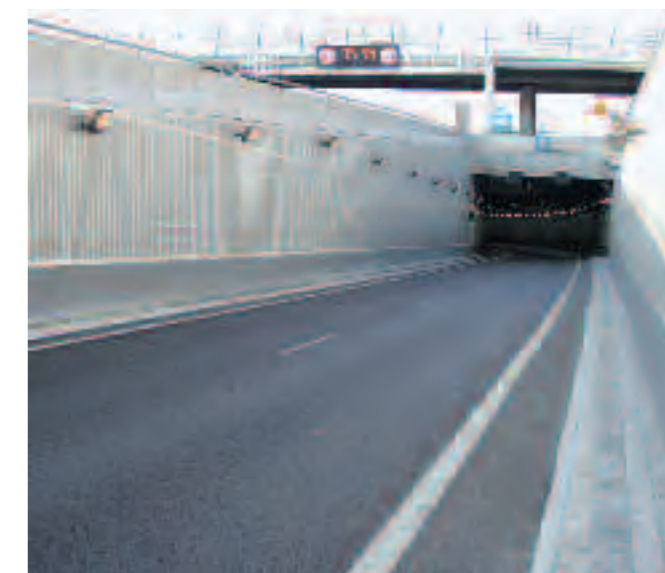
Túnel By-pass Sul, Madrid.
