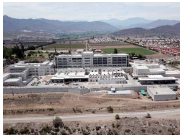
Hospital de Ovalle (Chile)
