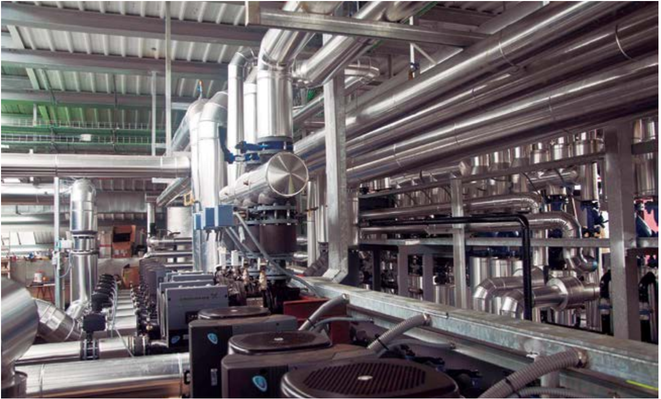
■ Electrical works of the Terminal Building of the Airport of Vigo
