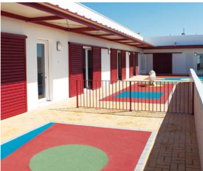
■ Victoria Kent Nursery School in Osuna, Seville
