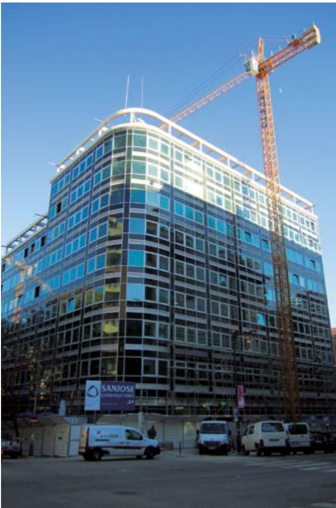
■ Refurbishment of an Administrative Building at 24, Castilho, Lisbon (Portugal)
