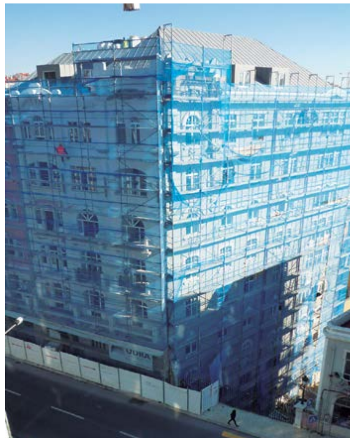
■ Refurbishment of the 4* H10 Hotel, Lisbon
