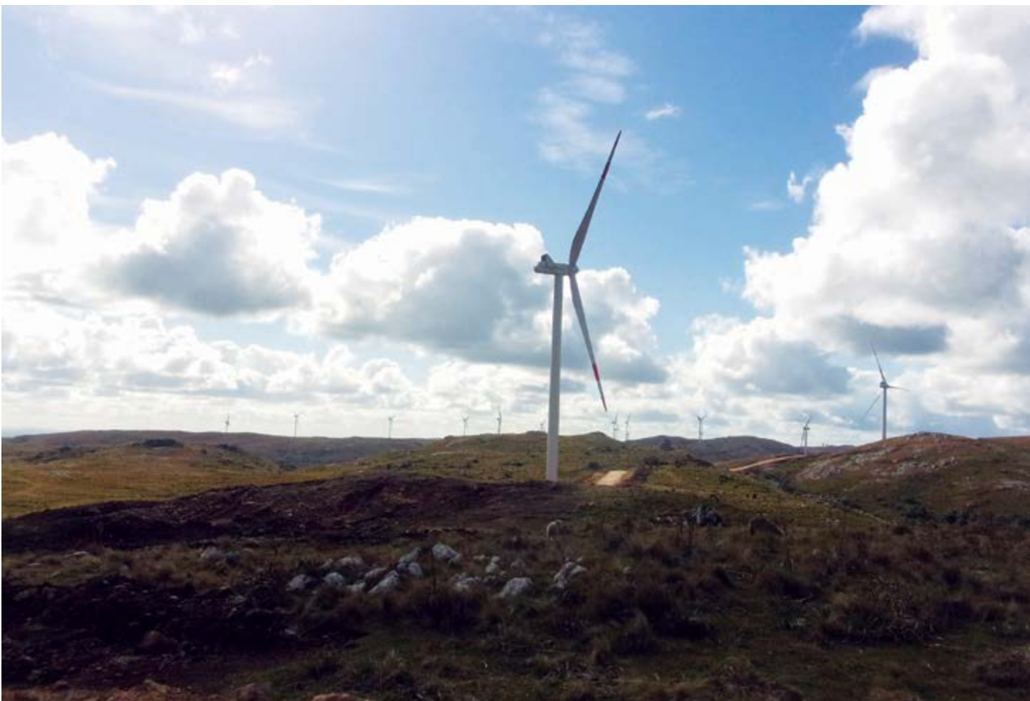
■ Wind farms in Uruguay (90MW) Engineering and project: GSJ Solutions / Execution: SANJOSE Constructora
