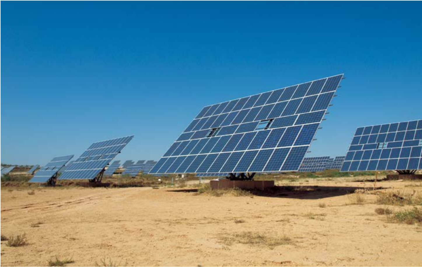
8.89 MW PV solar plant in Valtierra, Navarra
