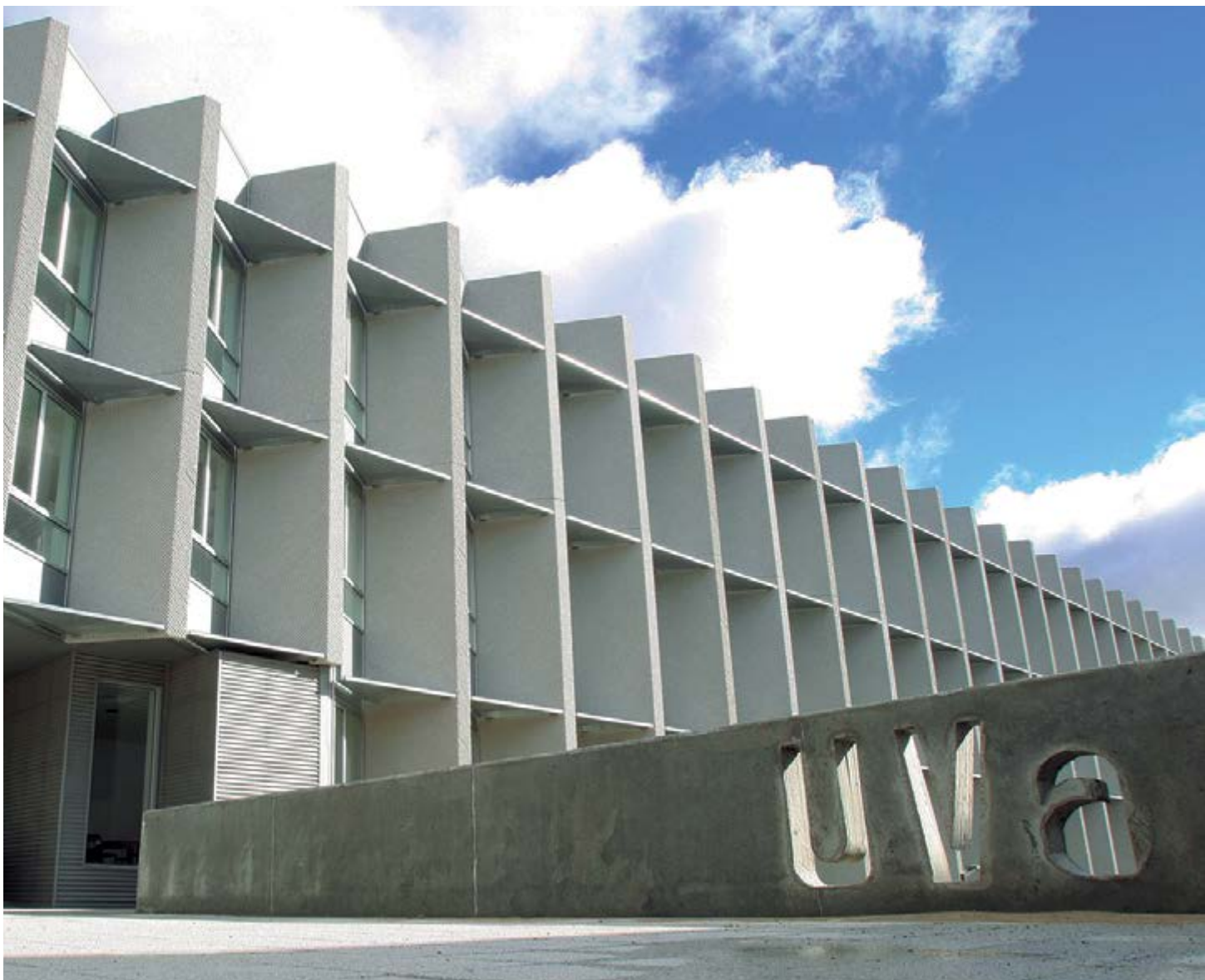
■ Building of the University Launching Platform for Applied Research Centres (LUCIA), University of Valladolid Certified with 98 Leed Platinum points as the most sustainable building of Europe and the second worldwide
