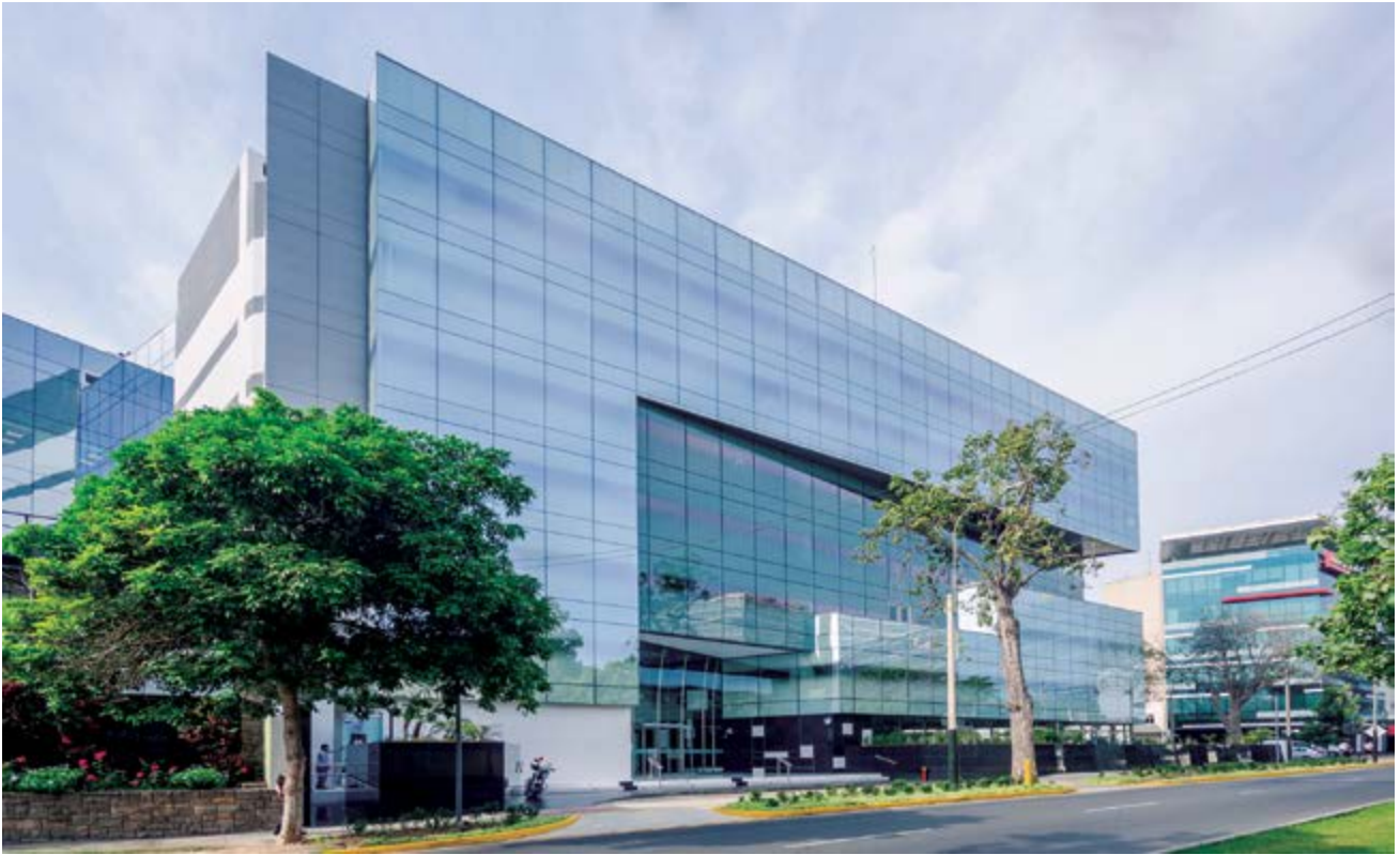
■ Administrative Building Av. Victor Andrés Belaunde, Lima (Peru)
