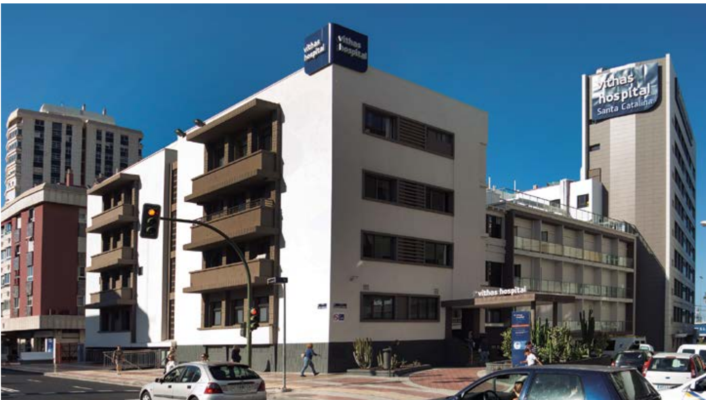
Refurbishment of the Vithas Santa Catalina Hospital of Las Palmas de Gran Canaria
