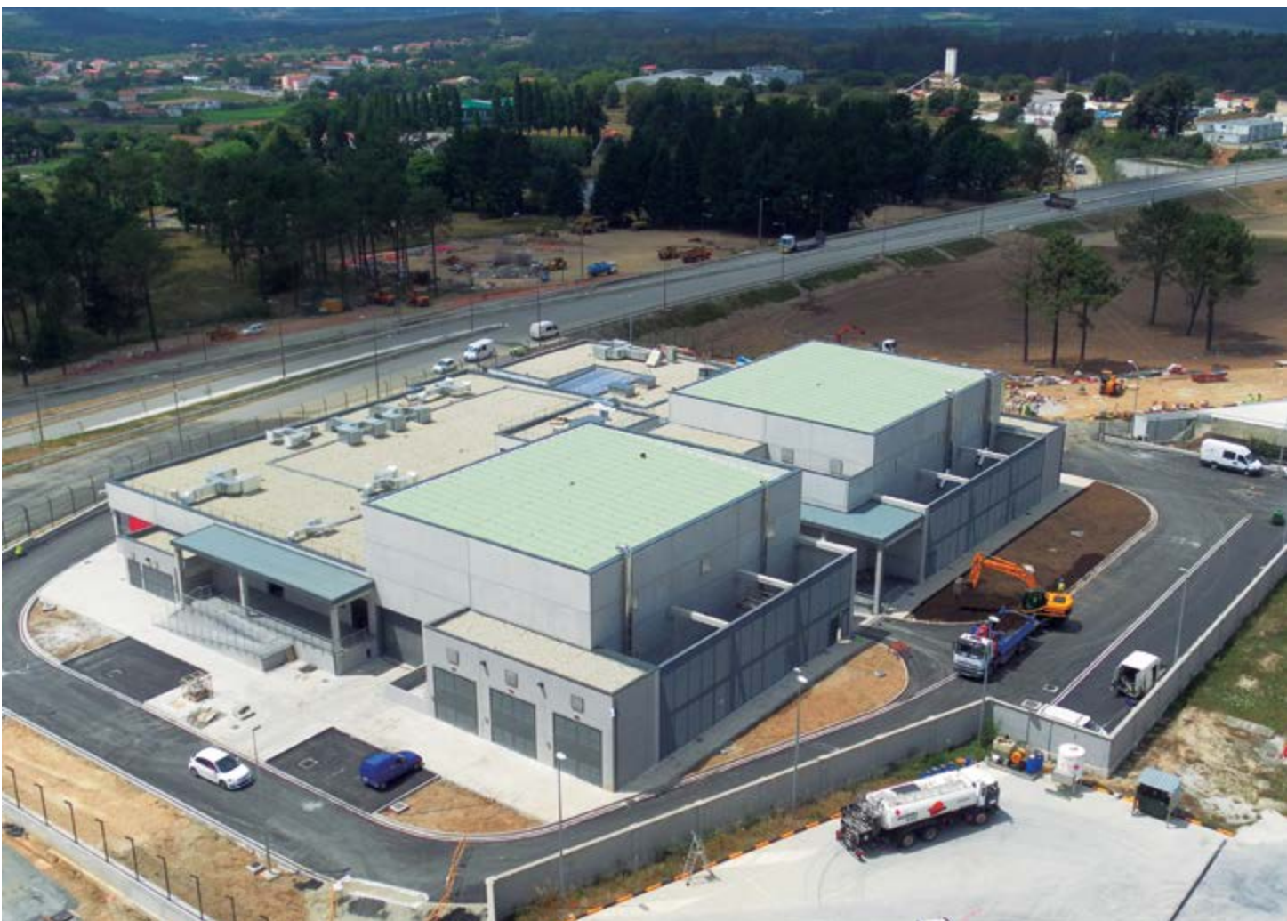
■ Electrical power station of the Airport of Santiago de Compostela
