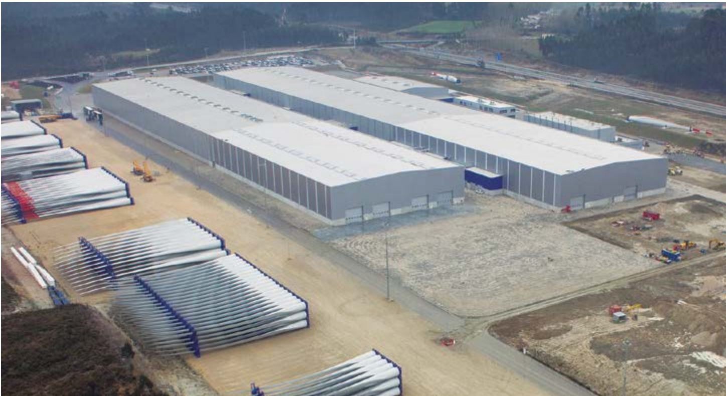
■ Enlargement of the factory of Ria Blades in Vagos, Aveiro (Portugal)
