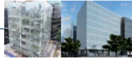
Tempus Administrative building, Lima
