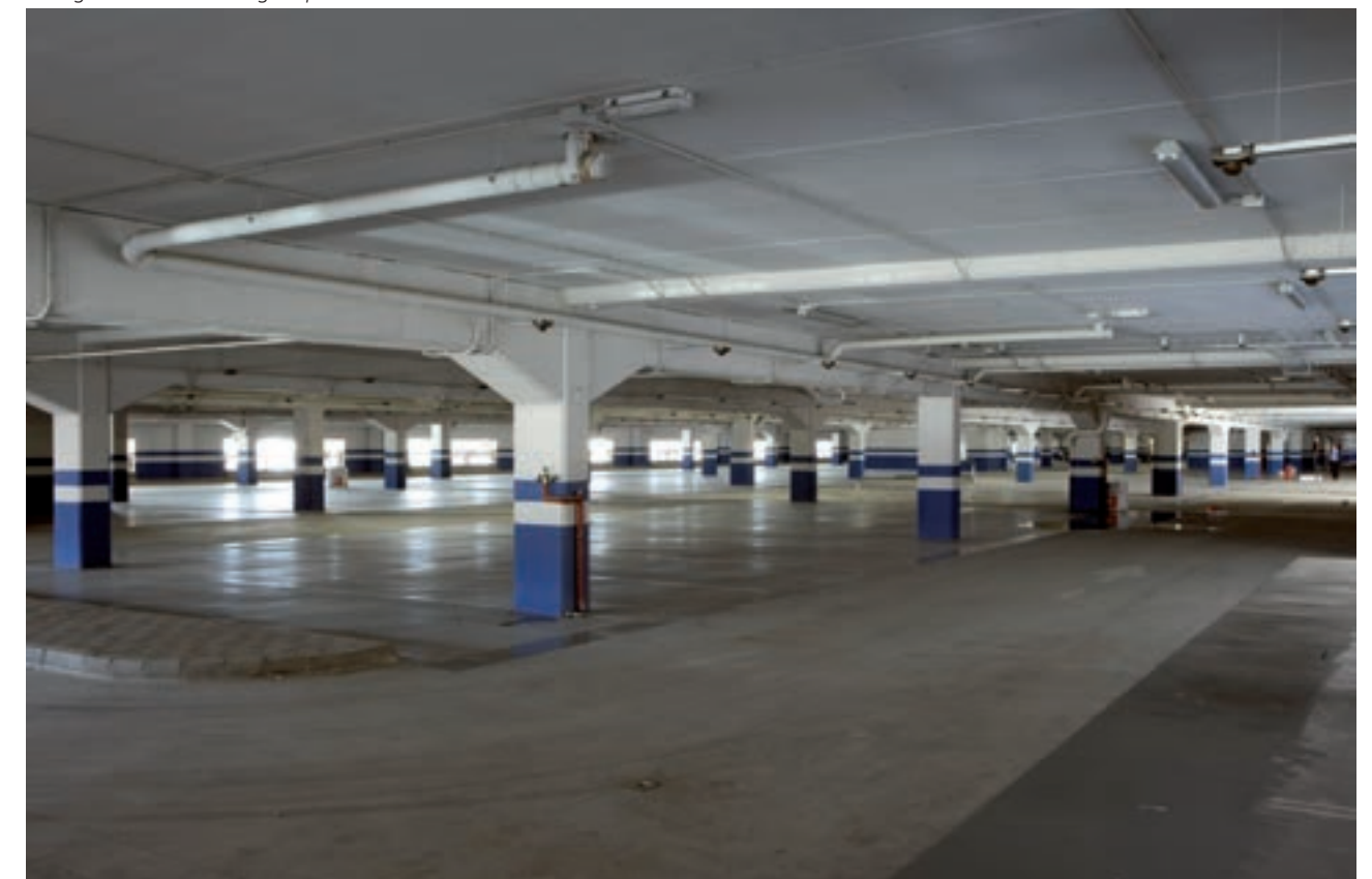
Parking structure at the Malaga Airport
