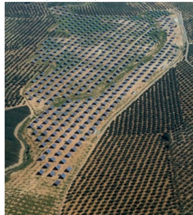
El Gallo electrical photovoltaic power plant of 5,4 Mw, Jaen
