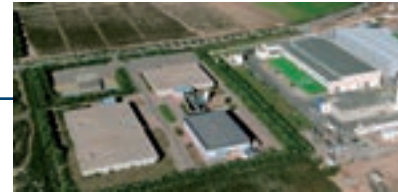
Extension of the Desalinization Plant in El Mojon, Murcia
