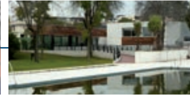
Municipal sport centre and swimming pool of Camas, Seville
