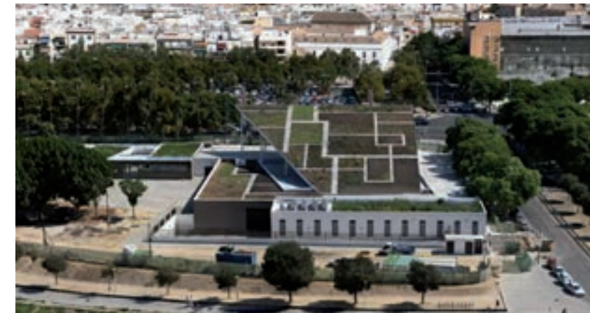
■ Restructuring of the former Cable Car Terminal of Expo 92 in Seville and execution of annex buildings for its restructuring into an Auxiliary Clean - up Park and sport facilities Land total surface. 5,240m 2 Gardens. 3,100m 2 , 1,600m 2 (1st at Seville) included Water sheets. 900m 2 Tiled floor 1,600m 2 Reusable fluvial water system Architect. Manuel Naranjo Alpresa
