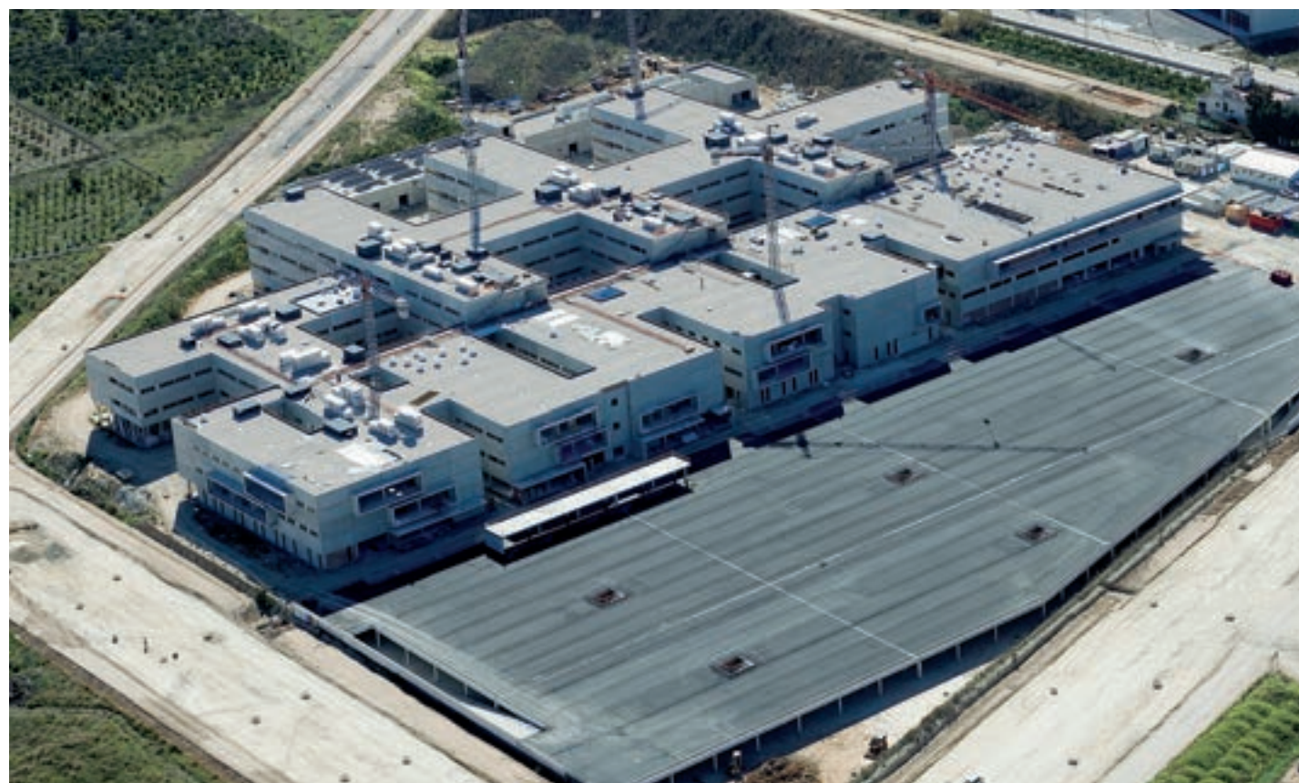
■ Hospital of Gandia Land total surface. 69,213m 2 Total surface. 48,640m 2 Total beds. 396 Intensive care units. 14 Surgery rooms. 10 Car park spaces. 530 Architects. Juan Añón Gómez, Gema Martí Sanjuán, Ramón Calvo Soto and José Ramón Tormo Illanes (AIC EQUIP Arquitectos & Ingenieros)
