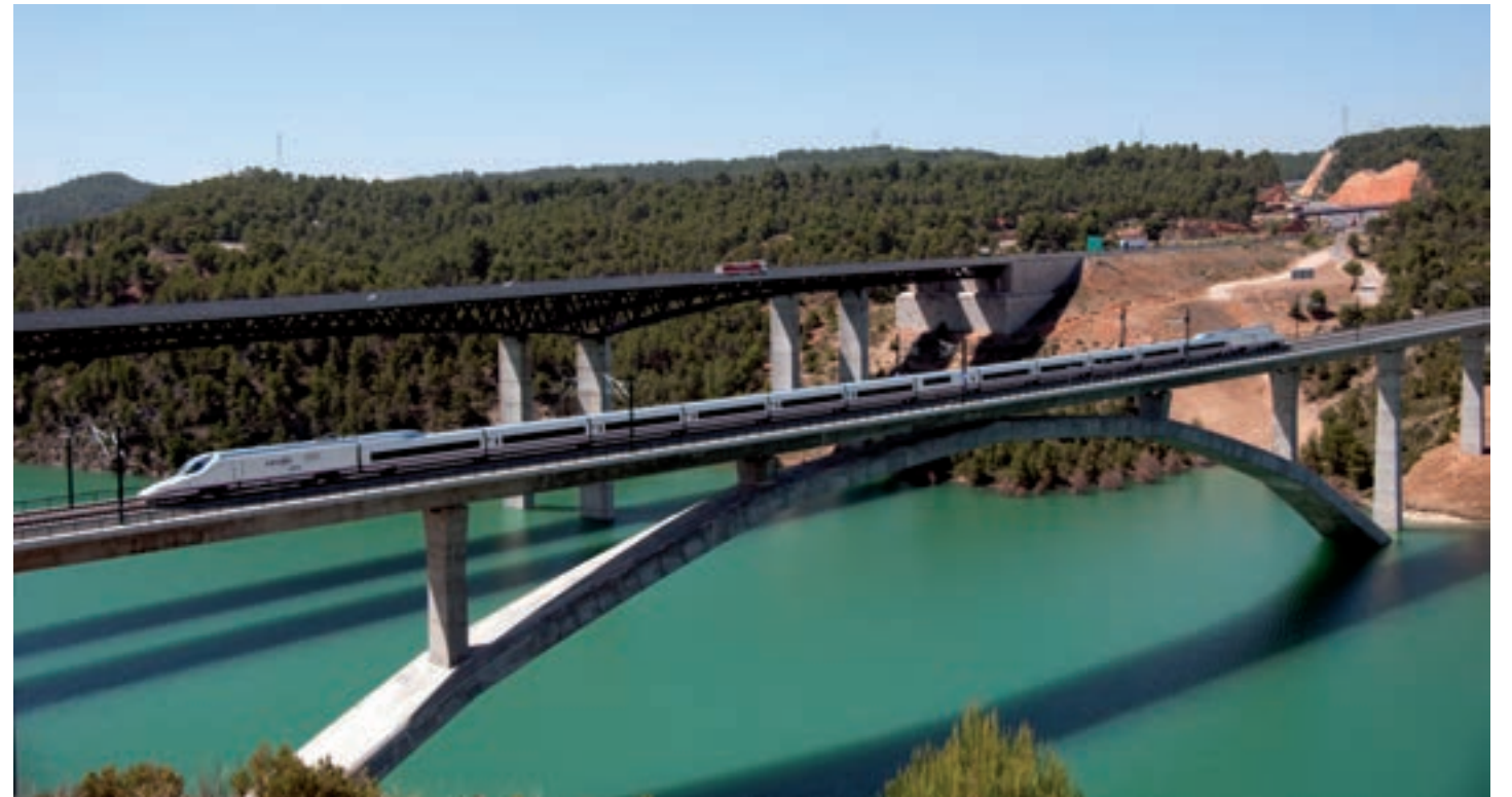
■ Strech Contreras Reservoir - Villargordo del Cabriel. Spanish National High speed Railway Network (AVE) Madrid - Valencia Length. 6.5 km Viaducts. 3 Tunnels. 3 Viaduct of Contreras. Greatest concrete railway arch in Europe and Spain (261 m span) Puente de Alcántara International Award
