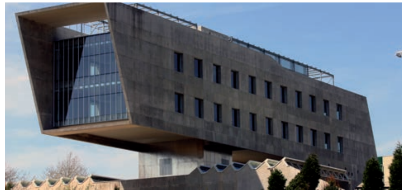
Research and Technology Building of the University of Vigo
