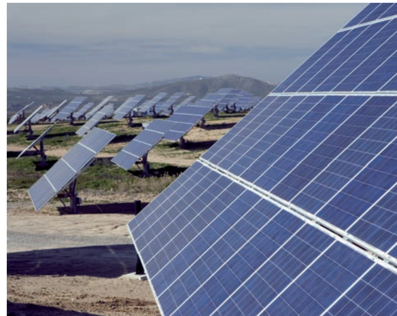
Photovoltaic Solar Energy
