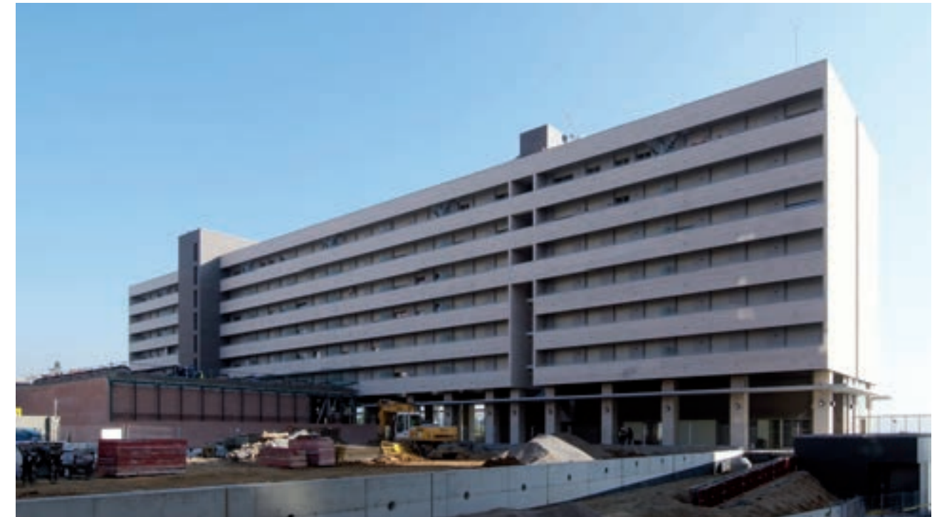
Social housing units and Public Municipal Library in Cornella de Llobregat, Barcelona
