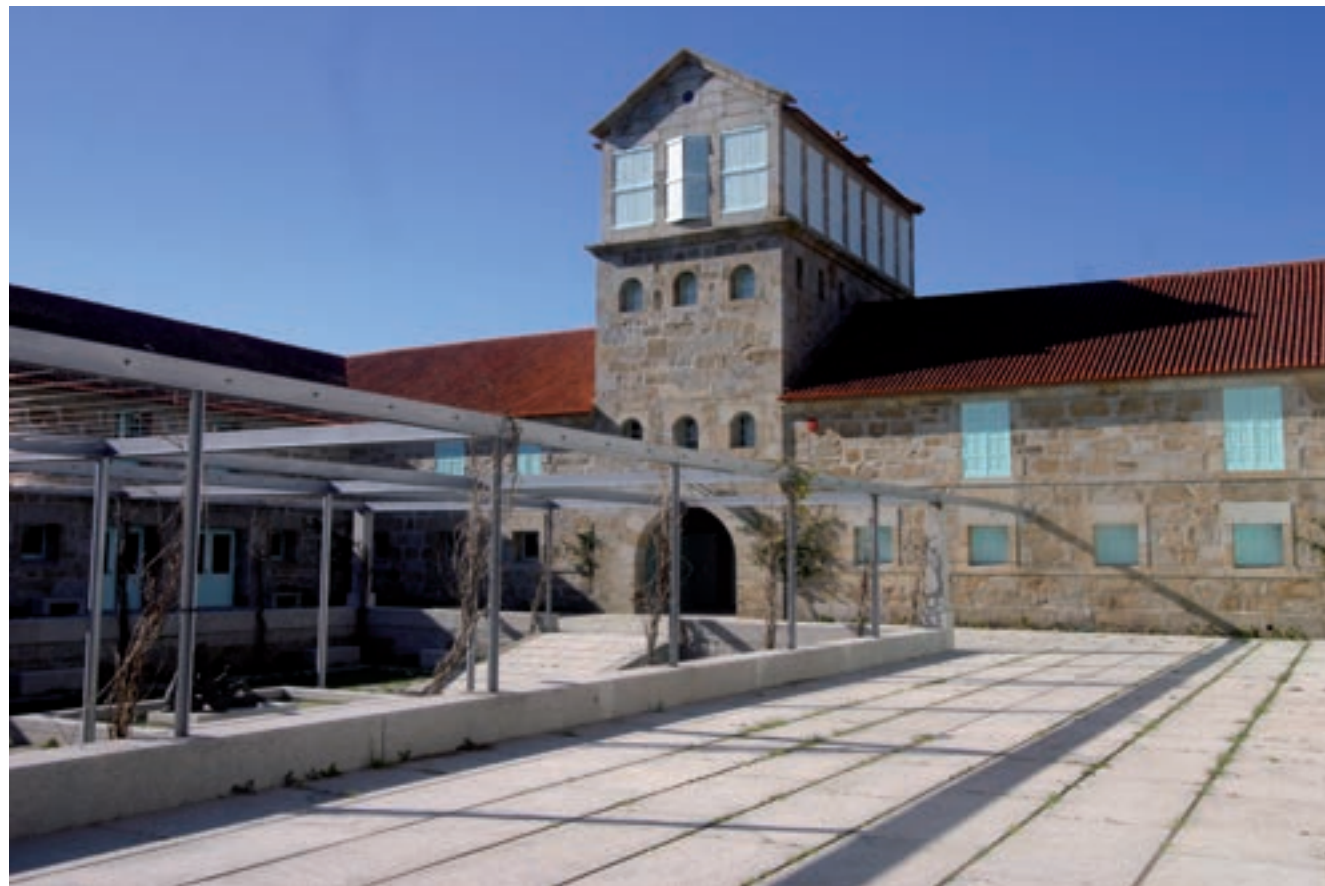
Rehabilitation of "Pazo Baion", Pontevedra
