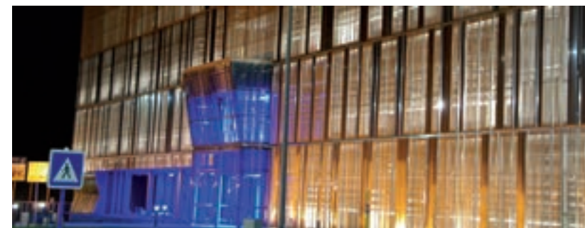
■ "Energigune" Research Centre at the Technology Park of Miñano, Alava Land total surface. 5,847m 2 A level energy coding. Use of alternative heating systems, such as biomass, geothermal and solar panels and photovoltaic Building characterised by the use of stainless steel screens which reflect the environment Architect. Javier Aja Cantalejo - ACXT (Idom)
