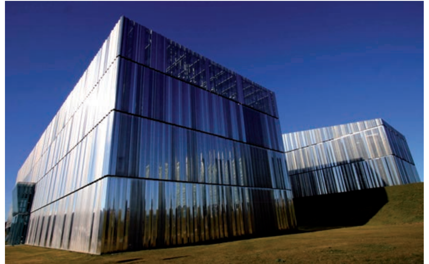
■ "Energigune" Research Centre at the Technology Park of Miñano, Alava Land total surface. 5,847m 2 A level energy coding. Use of alternative heating systems, such as biomass, geothermal and solar panels and photovoltaic Building characterised by the use of stainless steel screens which reflect the environment Architect. Javier Aja Cantalejo - ACXT (Idom)
