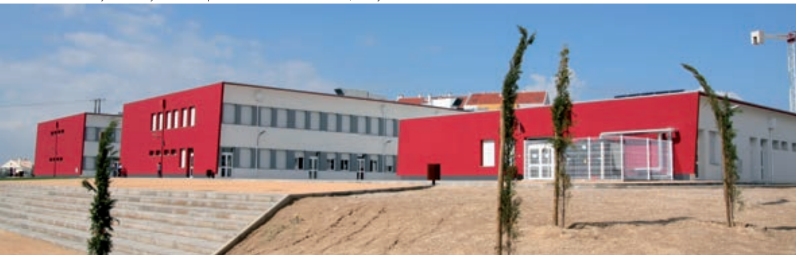
Nursery and Primary School and Sports Pavilion of the Barrio de Areias, Montijo
