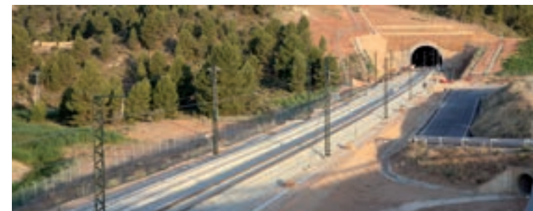
■ Strech Contreras Reservoir - Villargordo del Cabriel. Spanish National High speed Railway Network (AVE) Madrid - Valencia Length. 6.5 km Viaducts. 3 Tunnels. 3 Viaduct of Contreras. Greatest concrete railway arch in Europe and Spain (261 m span) Puente de Alcántara International Award
