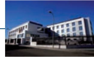
Arenas Hotel in Pinto, Madrid
