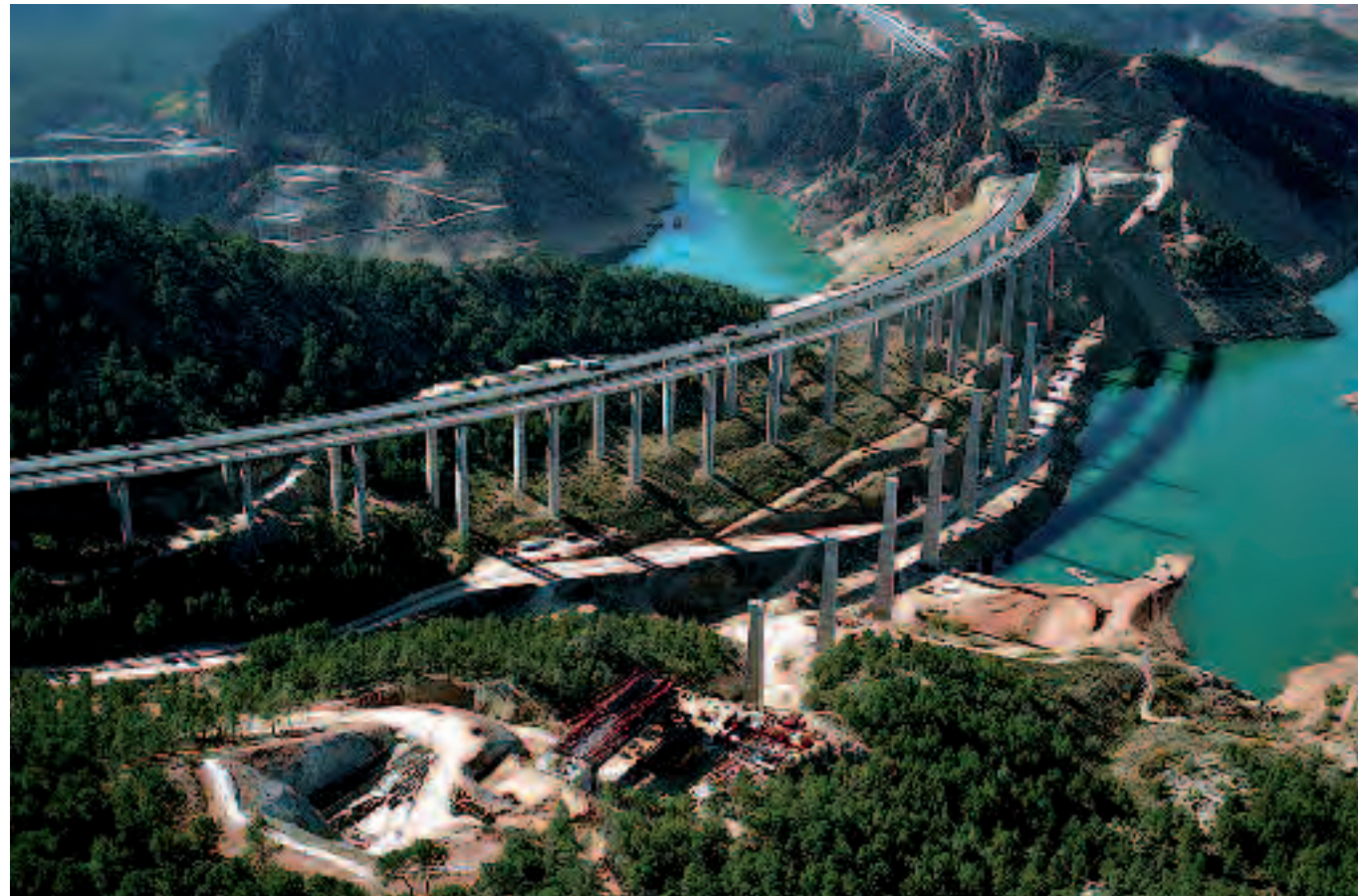
High Speed Railway Madrid-Valencia Line.
