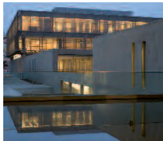
Trigeneration in the Provincial Council of Málaga.
