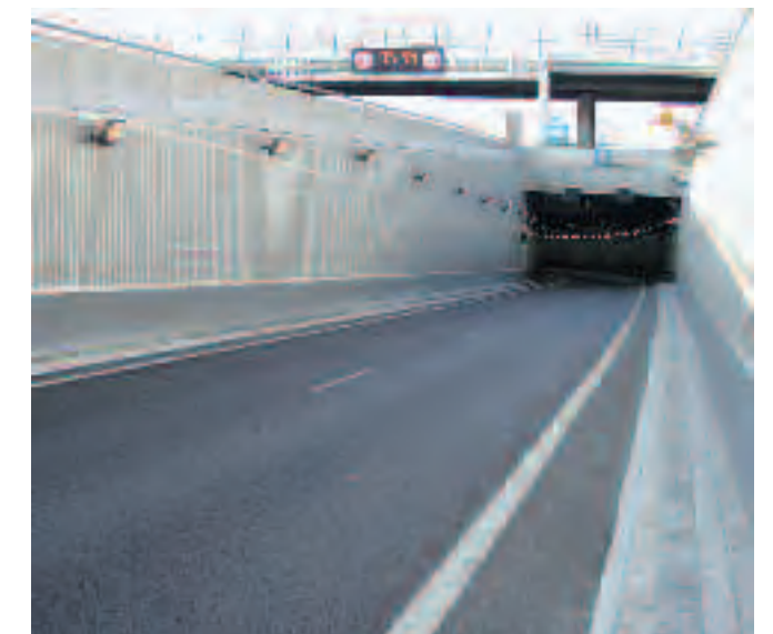
Tunnel By-pass South / M-30, Madrid.
