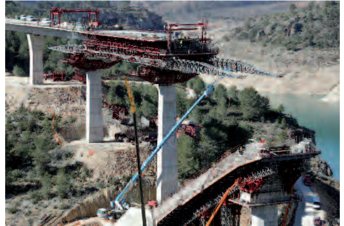
High Speed Railway Madrid-Valencia Line.
