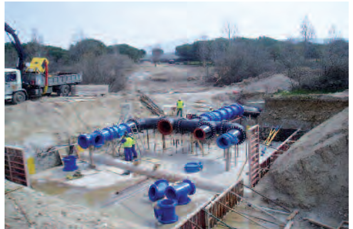
Water Supply Systems to Manzanares el Real, Madrid.
