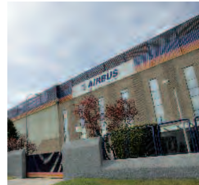
AIRBUS Production Plant in Illescas, Toledo.
