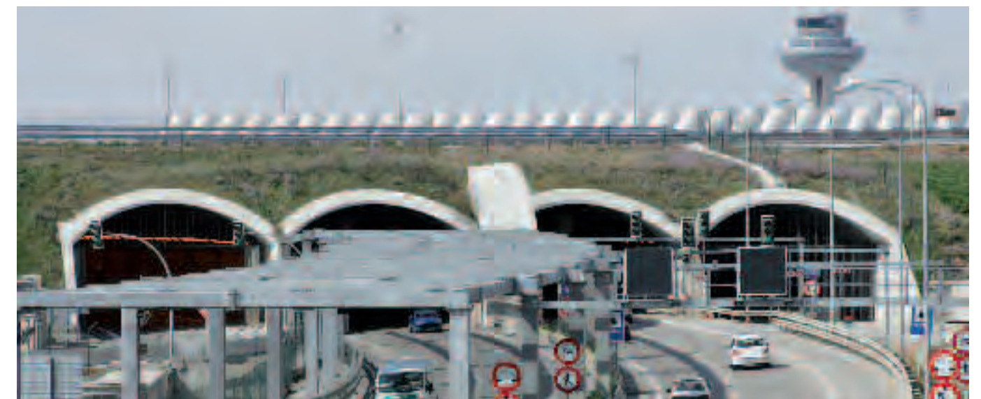
Tunnels from Barajas Airport, Madrid.
