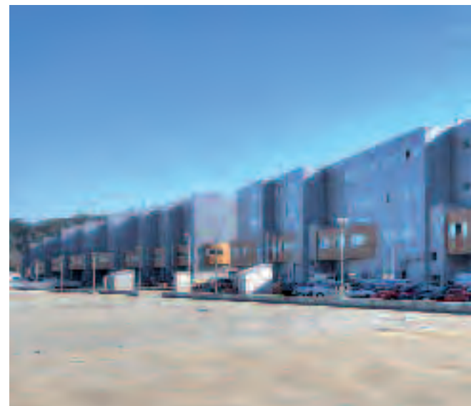
Texvigo Industrial Buildings, Pontevedra.
