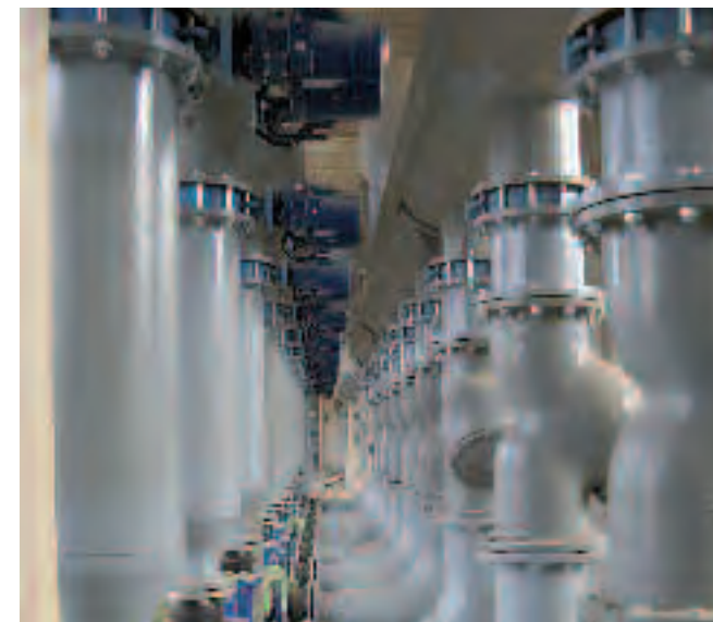
Power Plant at the Airport of Barcelona.
