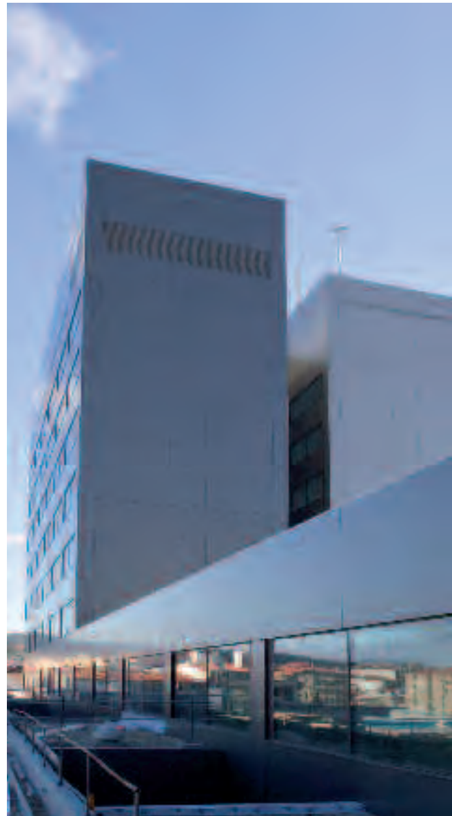
Administrative Building for the Government of Galicia in Campolongo, Pontevedra.
