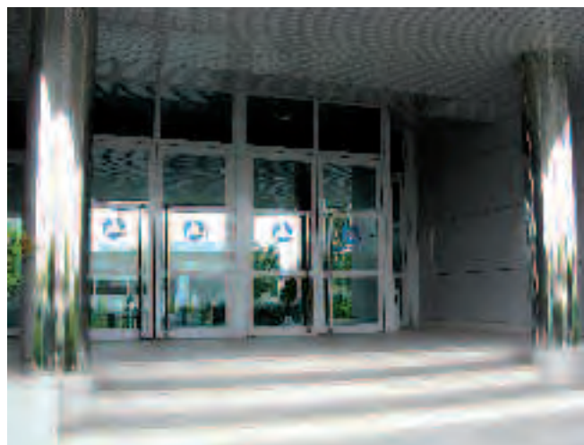
Central Headquarters of SANJOSE in Tres Cantos, Madrid.
