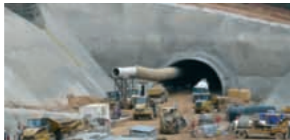
High Speed Railroad access of Madrid-Valencia.
