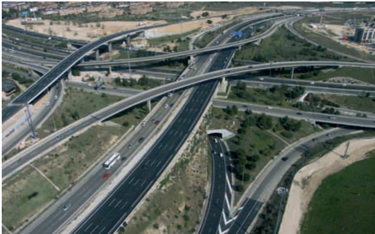
Junction of Las Tablas with the M-40, Madrid.
