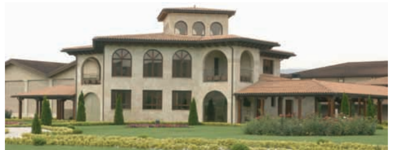
Main building of the Altanza Winery in Fuenmayor, La Rioja.
