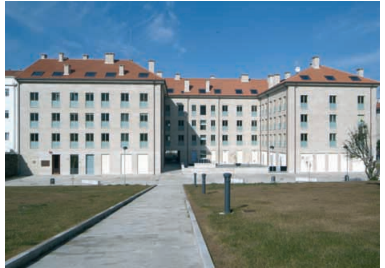
Residential development Las Galeras, Santiago de Compostela.
