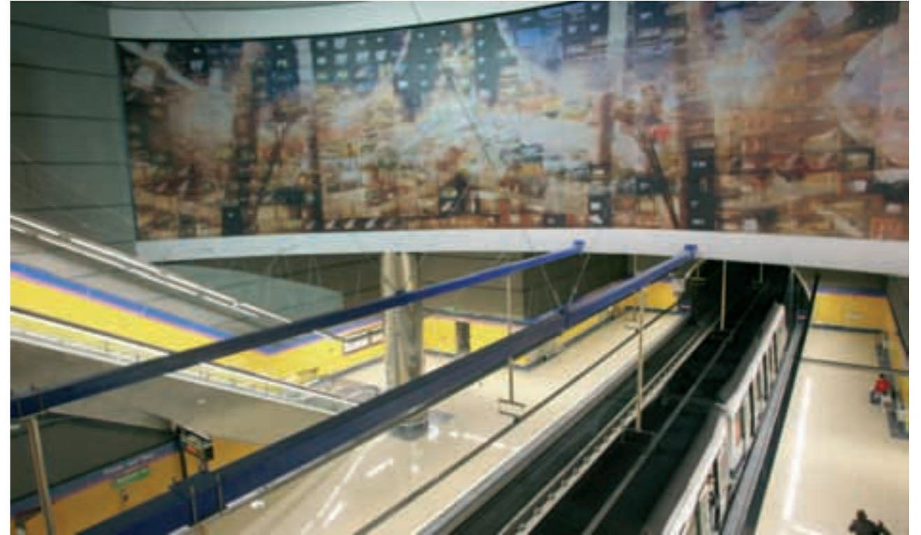
Metro station Pinar del Rey, Madrid.
