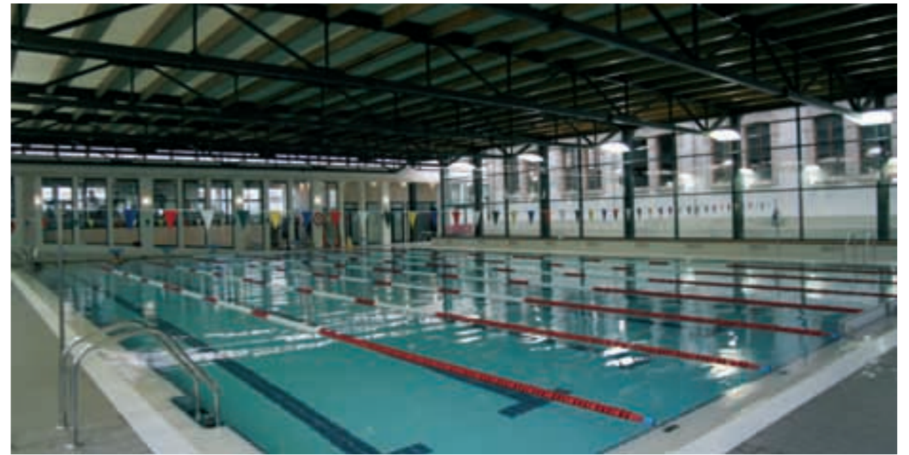
Indoor Swimming Pool of Alcoy, Alicante.
