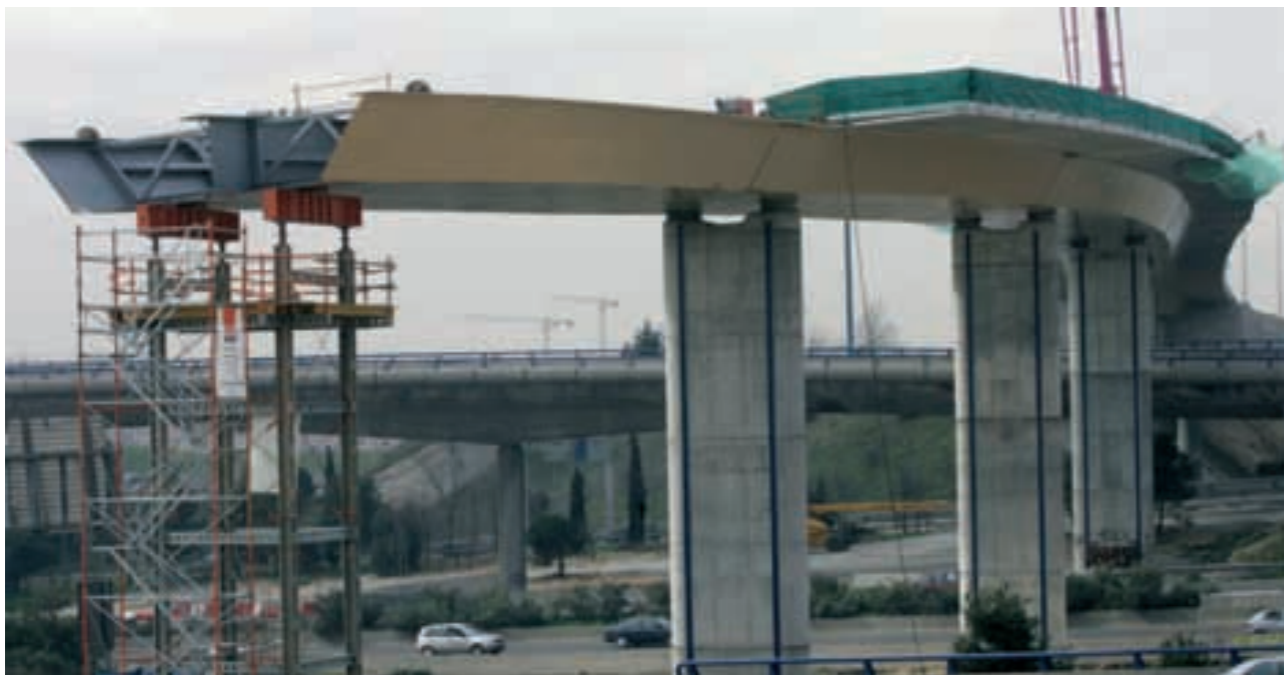
Junction of Las Tablas with the M-40, Madrid.
