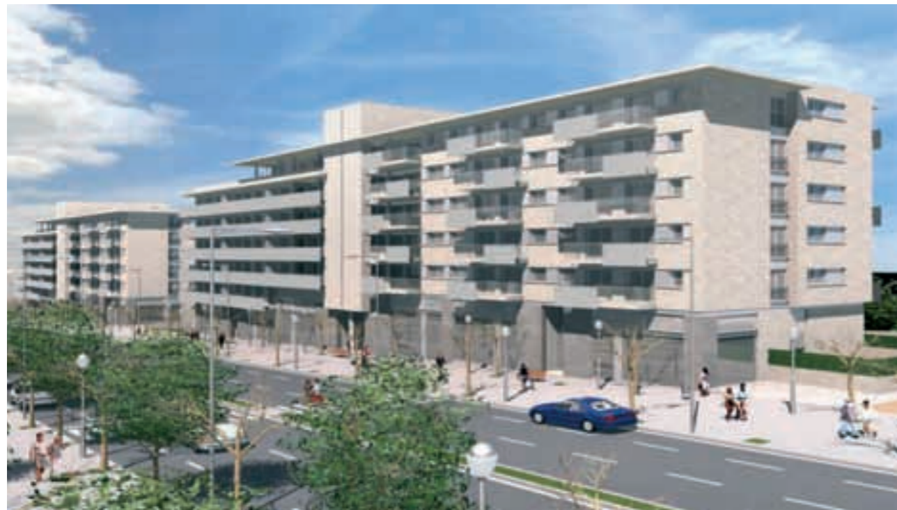
Residential development Espai Boulevard, Tarragona.
