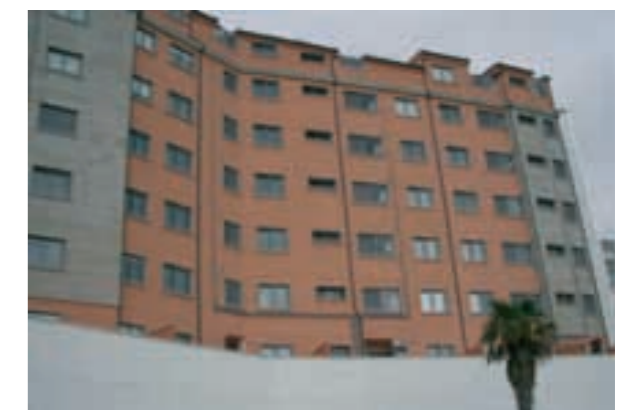
Residential development in Avda. de Vigo, Pontevedra.
