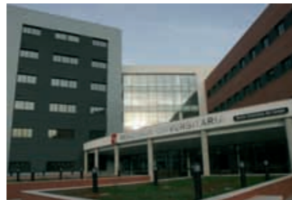
University Residence Hall "Heliópolis", Sevilla.
