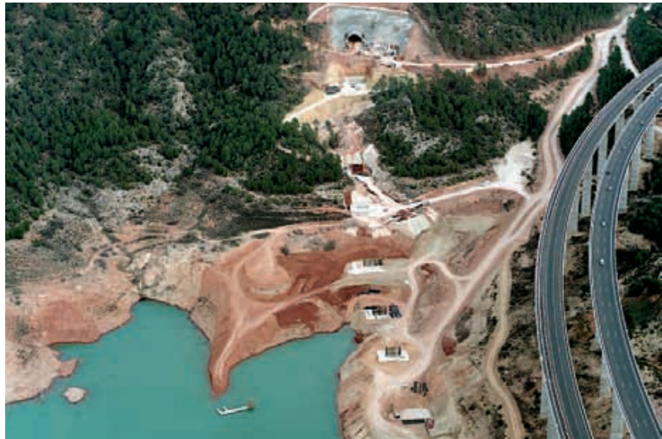
High Speed Railroad access of Madrid-Valencia.
