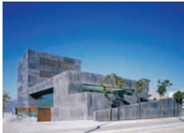
Courthouse of Antequera, Malaga.
