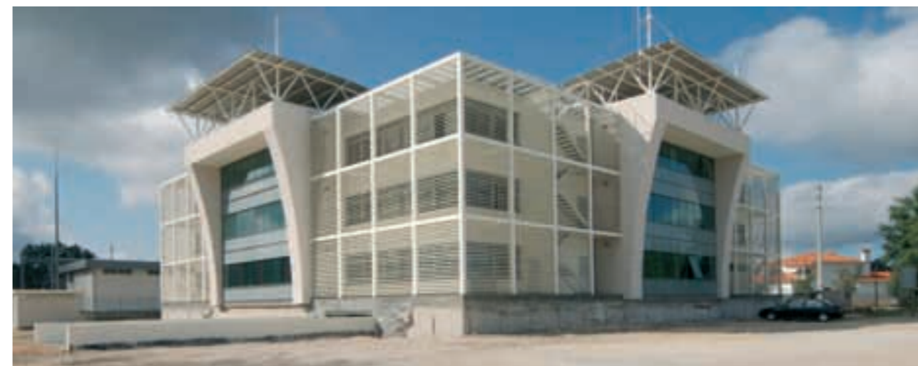
Main Office of Mira Businesses, Aveiro.
