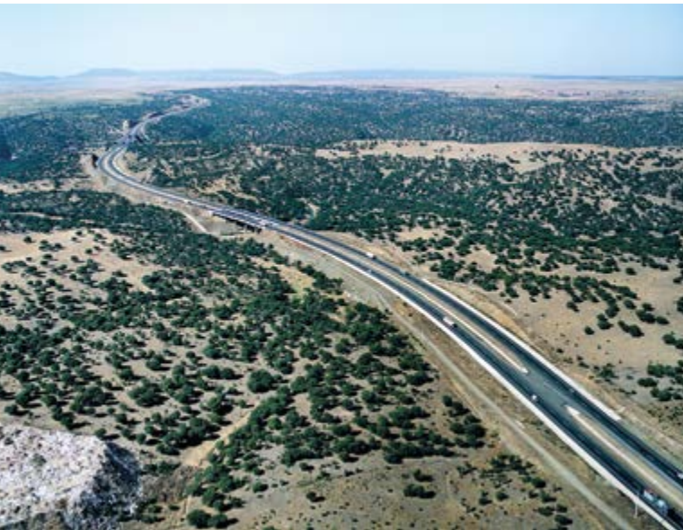
Conservation and operation of the state roads sector CC-0305 Cáceres, Extremadura (Spain)
