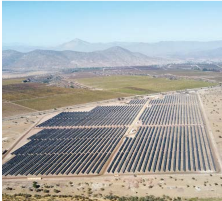
Los Nogales Photovoltaic Plant, Ovalle Region (Chile). 9.9 MW
