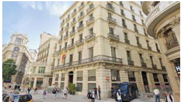
Directorate General Building of Police of Barcelona (Spain)
