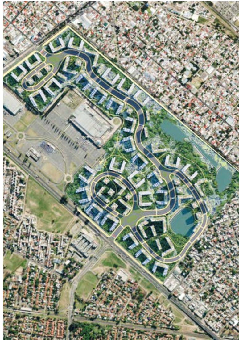
Urban Transformation La Tablada – 20,000 housing units-, Buenos Aires (Argentina)
