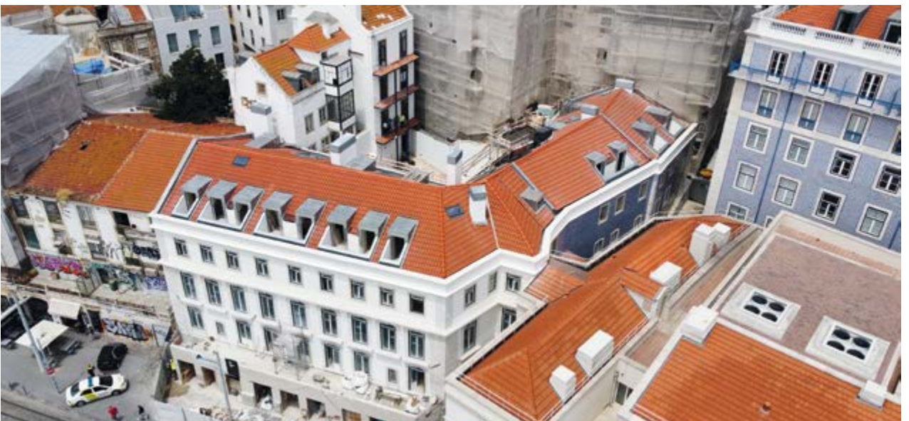
Campo das Cebolas 1-12 Residential Development, Lisbon (Portugal)
