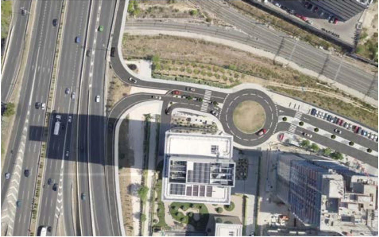
Access to the Manoteras Warehouses - Isla de Chamartín, Madrid (Spain)
