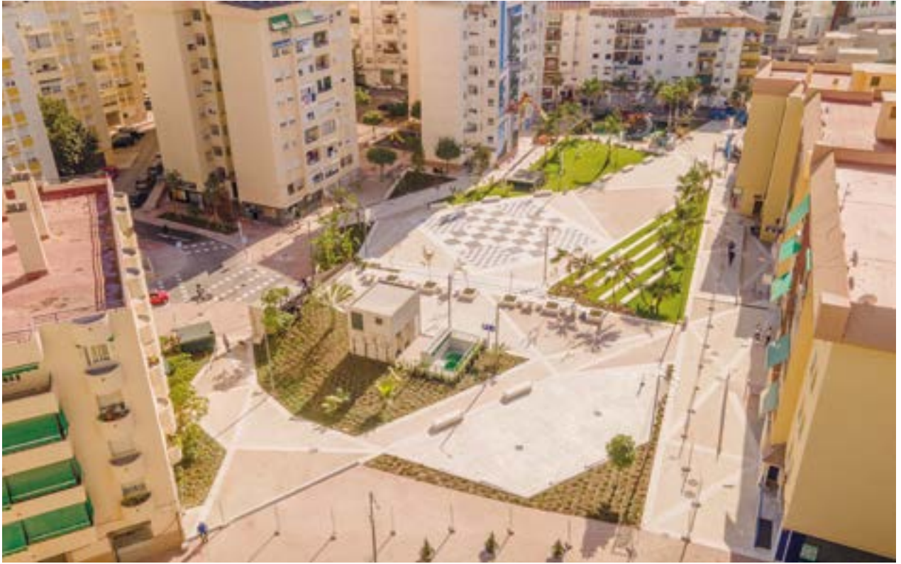
Underground parking in the Plaza del Ajedrez de Estepona, Malaga (Spain)
