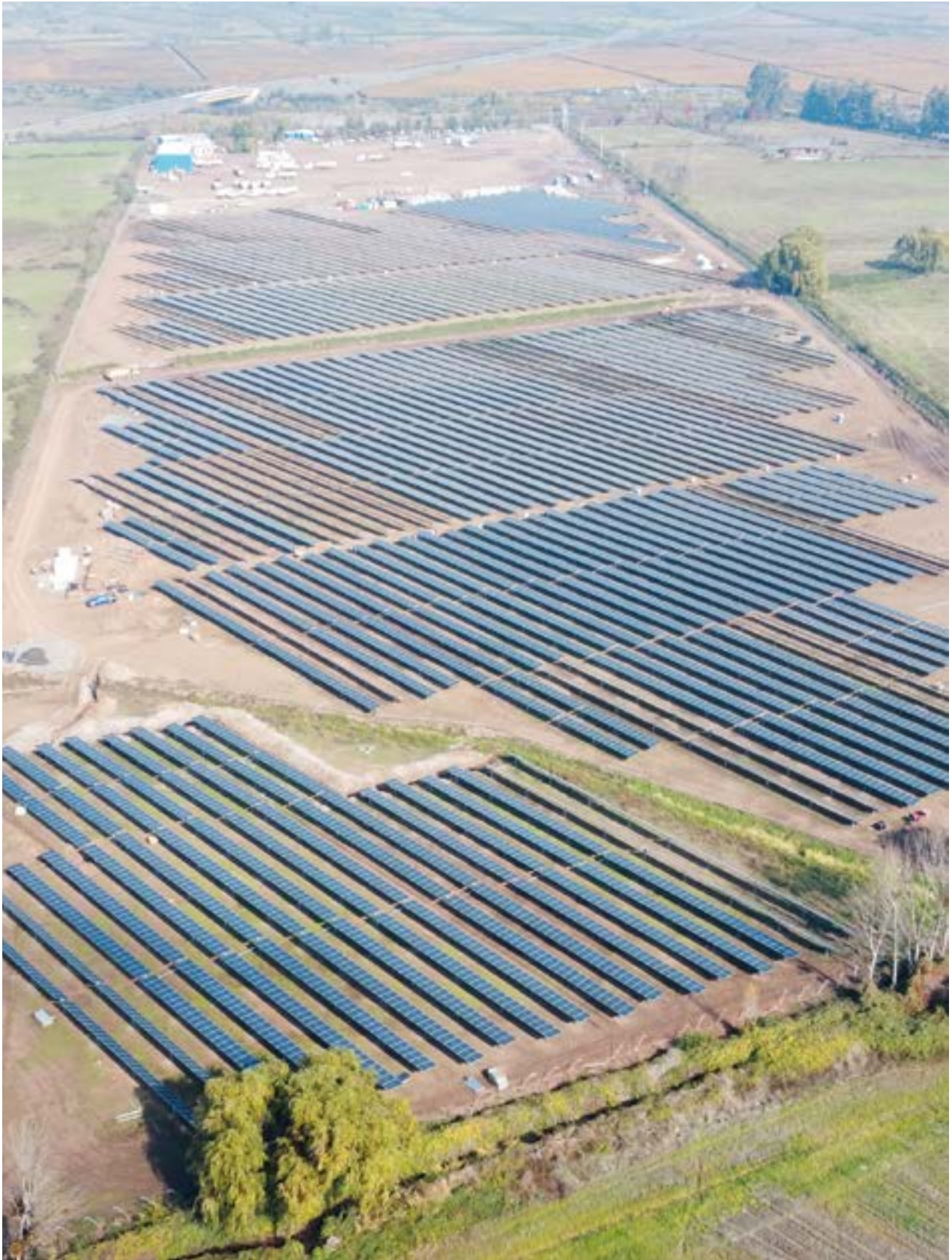
Milan Photovoltaic Plant, Maule Region (Chile). 7.36 MW
