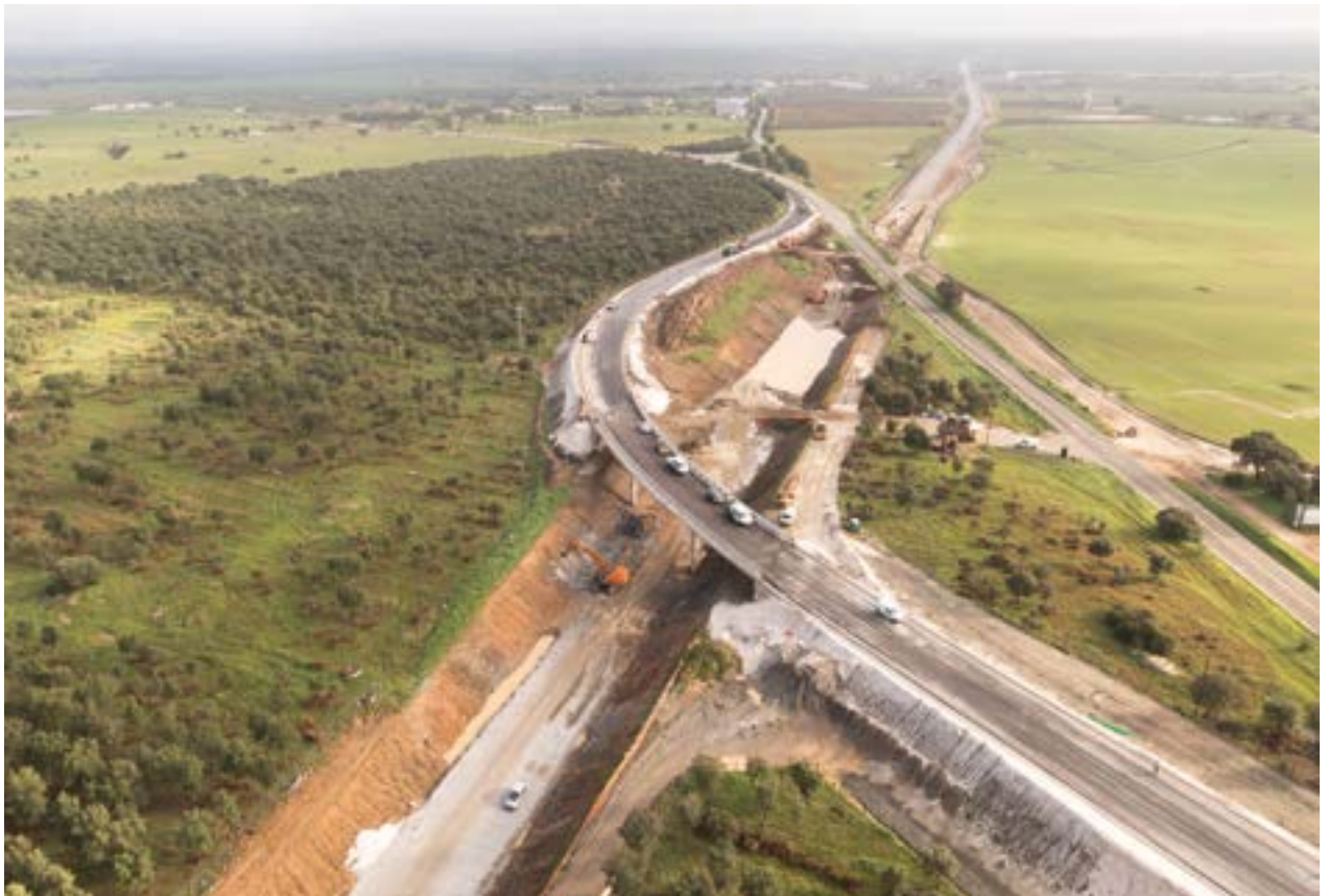
Stretch North Evora - Freixo of the Southern International Corridor (Portugal)
