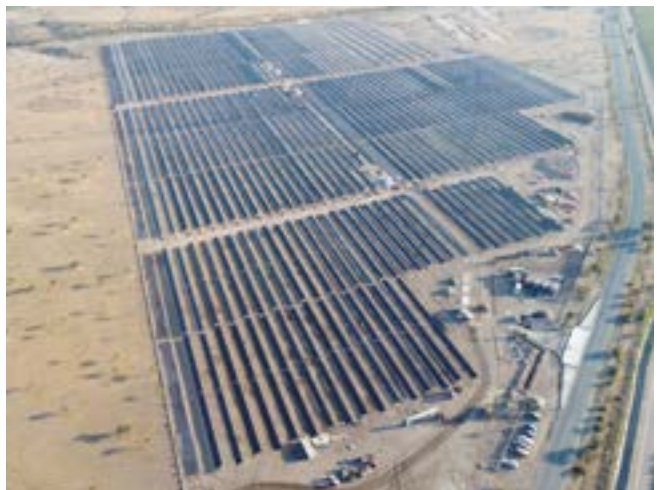
Los Nogales Photovoltaic Plant, Ovalle Region (Chile). 9.9 MW
