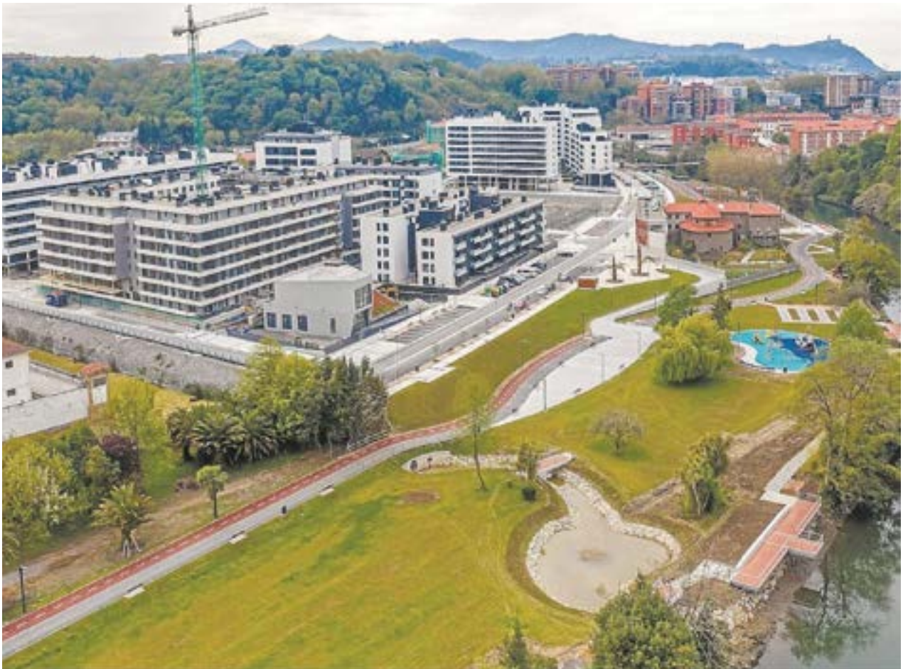
District Heating of the Txomin Enea eco-neighbourhood in Donostia - San Sebastián (Spain)
