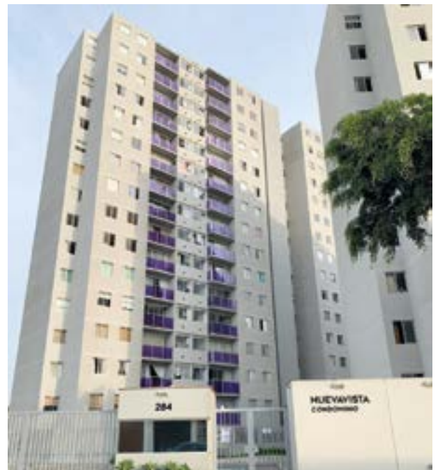
Nuevavista Condominium in the district of Bellavista in the Province of Callao 1,104 housing units-, Lima (Peru)
