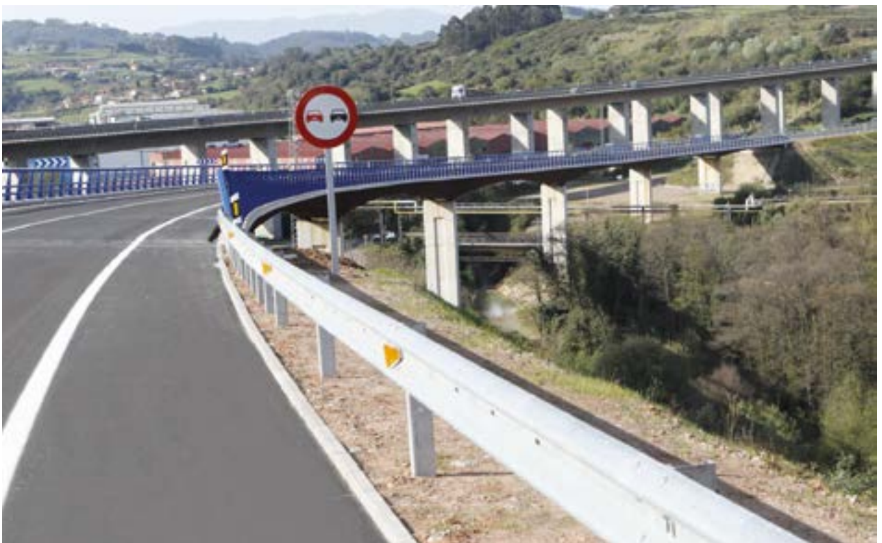
Access to the area of logistics and industrial activities of Asturias (Zalia) from the high capacity network (Spain)
