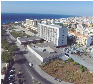
HEADQUARTERS OF THE CENTRAL BANK OF CAPE VERDE
