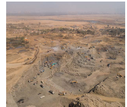
STRETCH 4 EARTHWORKS AND SOIL STABILISATION NEW AIRPORT NAVI MUMBAI.
