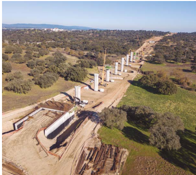
STRETCH ÉVORA NORTE - FREIXO OF THE SOUTHERN INTERNATIONAL CORRIDOR (PORTUGAL).
