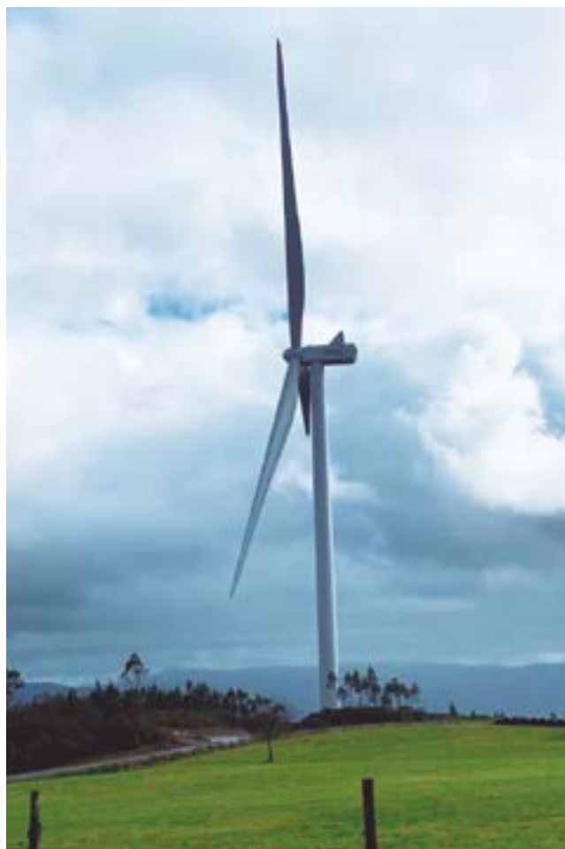
Wind farms for Norvento in Lugo (Spain)
