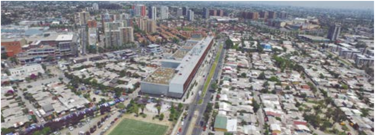
Metropolitan Hospital of La Florida, Santiago de Chile
