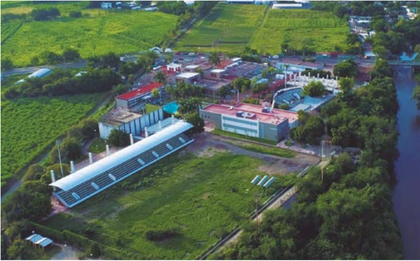
Refurbishment of the General Hospital Zone # 5 in Zapatec, State of Morelos (Mexico)
