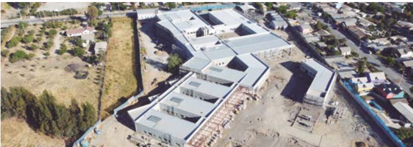
San José de Casablanca Hospital (Chile)
