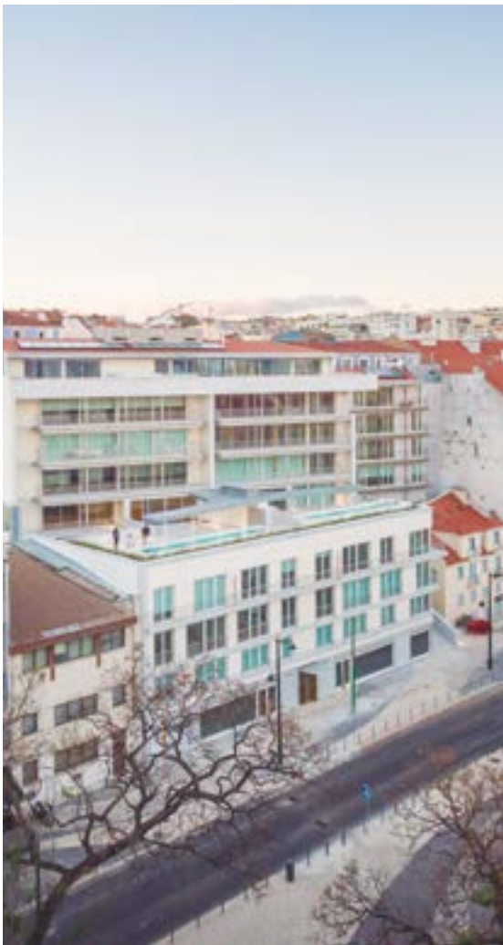
Santos Design Residential Complex, Lisbon (Portugal)
