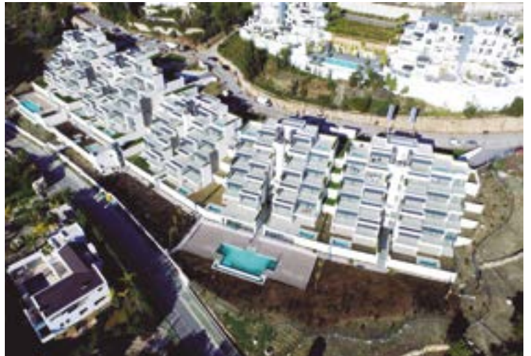
Aqualina Residential Complex in Benahavis, Málaga (Spain)
