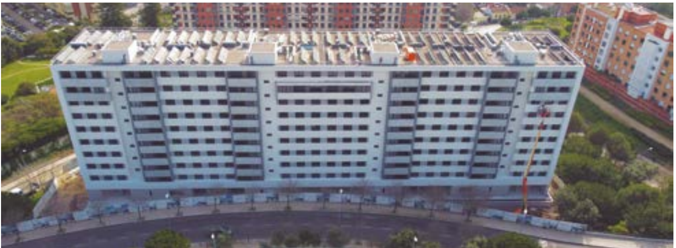
Residential Buildings at Almarjão, Mirafleres (Portugal)
