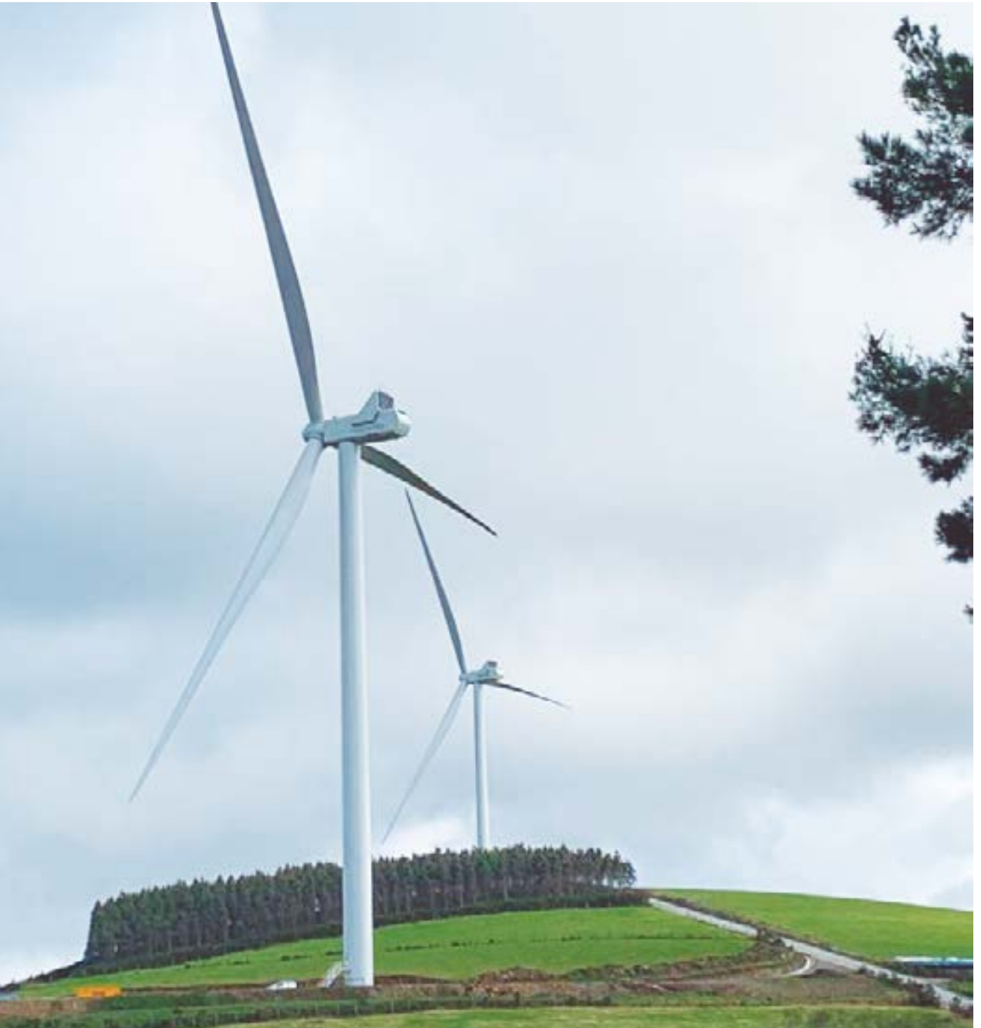
Wind farms for Norvento in Lugo of 65,7 MW (Spain)
