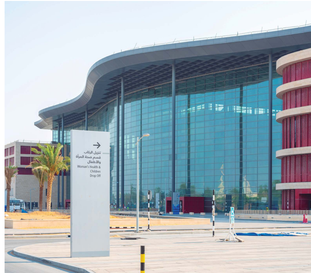
Al Ain Hospital, Abu Dhabi (UAE)
