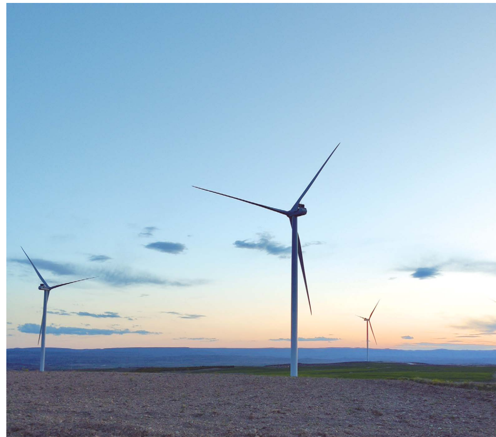
Wind farms for Enel Green Power in Teruel (176.6 MW)
