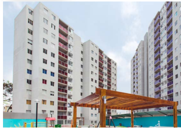
Nuevavista Condominium at the district of Bellavista in Callao, Lima
