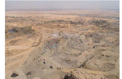
Stage IV earthworks and soil stabilisation New Airport Navi Mumbai
