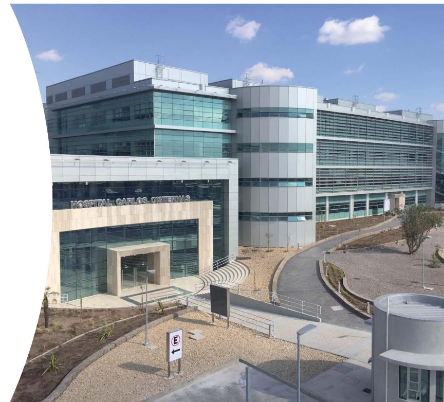
Carlos Cisternas Hospital, Calama (Chile)
