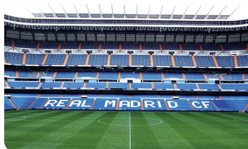
Santiago Bernabeu Stadium Maintenance of the Property of Real Madrid
